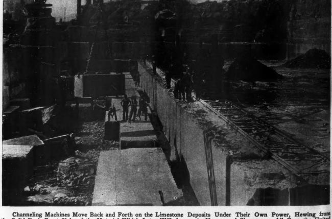
Channeling Machines Move Back and Forth on the Limestone Deposits Under Their Own Power, Hewing from the Solid Rock Great Slabs of the Material Which Later Will Appear in Homes and Skyscrapers All Over the United States.
