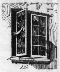
Outswinging Casement Windows Which Can Be Washed From Inside the House Are a Convenience Which Will Be Appreciated by the Housekeeper.
