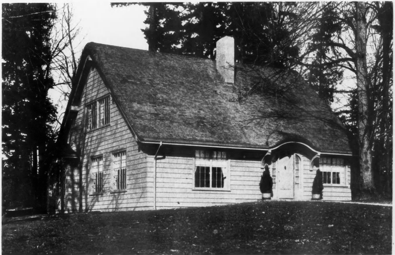
Shingles Rounded at the Eaves and Over the Arch of the Doorways Give to This Home a Delightful Air of Old World Snugness, Decidedly in Keeping With the Soft Tones of the Shingled Sidewalls. Full working details of this home will be found in the drawings on the four following pages.
