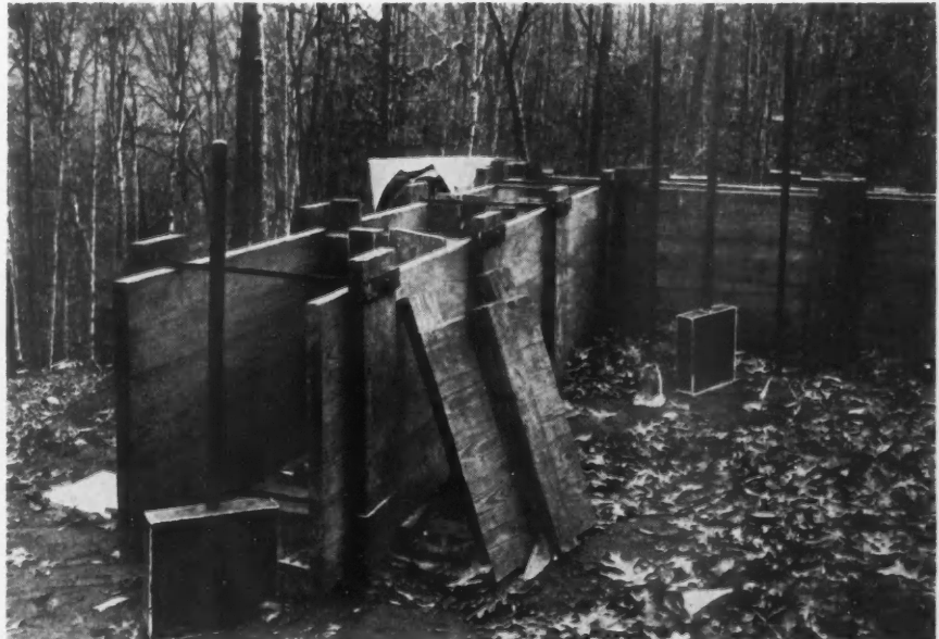
The Wooden Forms for Rammed Earth Construction Must Be Stronger than Those Used for Concrete. Notice in the picture the rams of different shapes.
