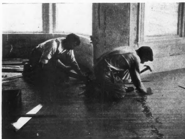
Laying 5/16-Inch Square Edge Oak Flooring.
