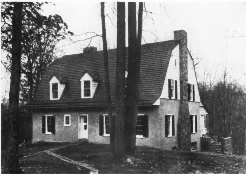
This Home with Walls of Rammed Earth, Recently Erected in Washington, D. C., Revived a Method of Building Used During the Time of Hannibal.
