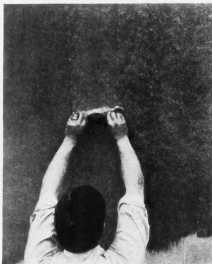
This Photo Shows How a Two-Tone Effect Is Produced by Using Paper Crumpled Into an Elongated Wad. After the ground color is dry the finishing color is applied and portions of the wet paint are lifted off by the paper allowing the ground color to show through.
