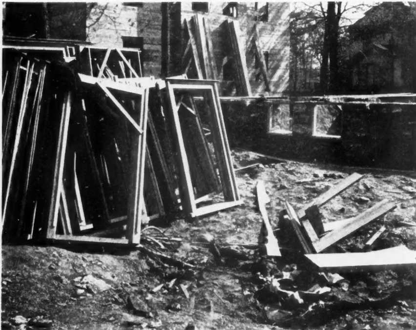
Unpainted Millwork Absorbs Moisture and Is Liable to the Attack of Wood-Destroying Insects. Rains may come, ground water may be absorbed or moisture from drying masonry or plaster may be taken up. Either moisture or insects will quickly destroy woodwork and the owner will blame the builder for costly replacements. A builder is manufacturer, merchant and consultant in one and, therefore, particularly in need of the good-will of his customer.
