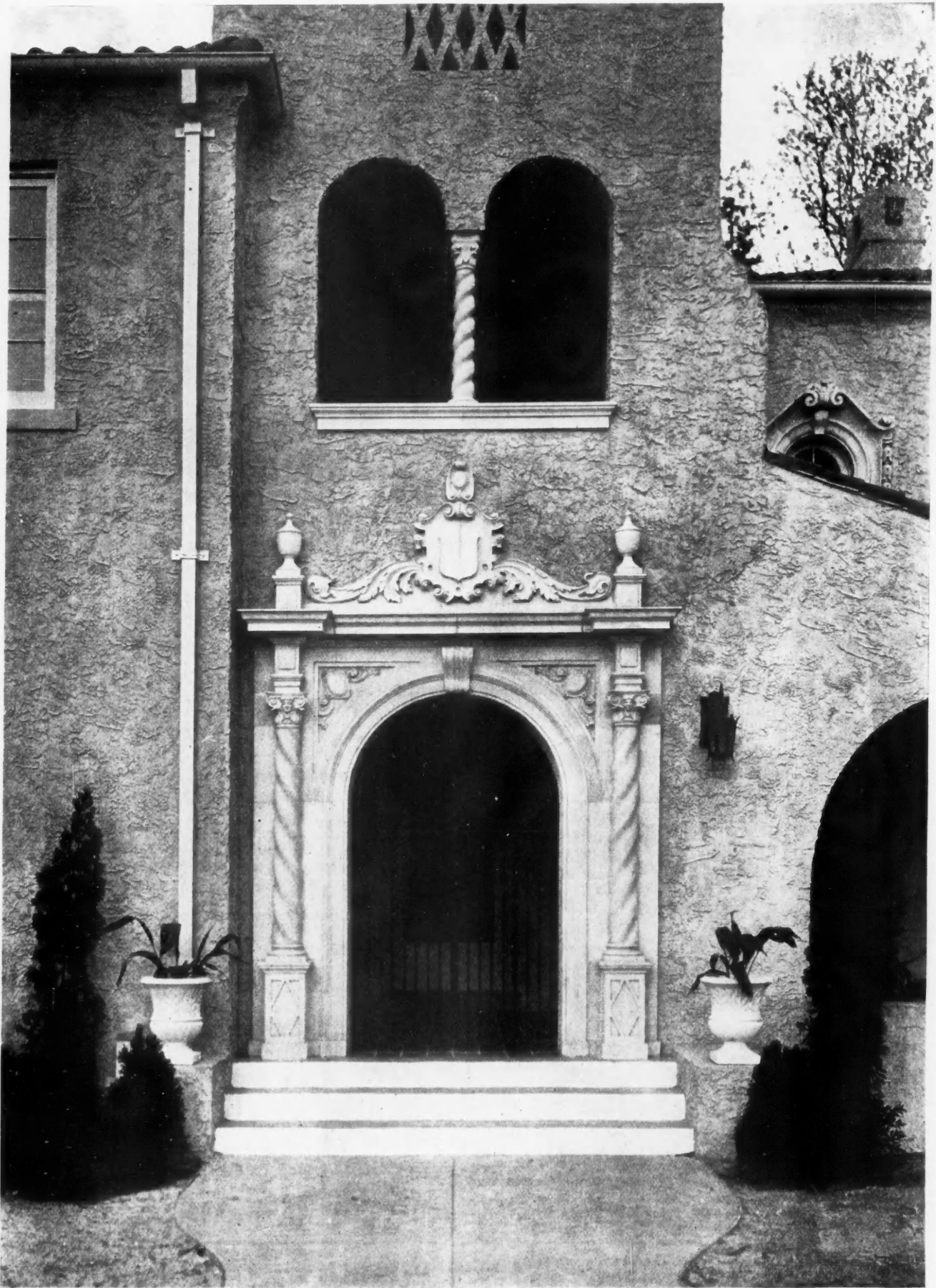
Careful Attention to Detail, as Revealed in This Doorway of the House Shown on Page 65, Has Been a Large Factor in Insuring the Ready Sale of the Homes Built by Telfair Stockton. The illustration shows plainly the interesting texture given to the stucco wall surfaces.
