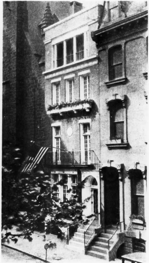
The Services of an Architect and Builder Were Sought and the Formerly Drab Exterior Was Transformed Into a Bright Spot in the Neighborhood.
