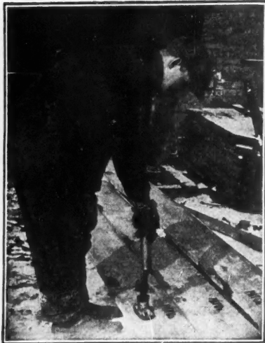
A Convenient Means of Marking Equipment Is Provided by a Self Heating Branding Tool.
