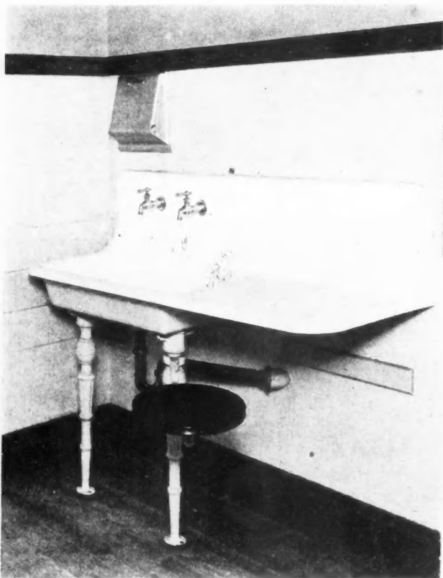
Just Below the Moulding in This Illustration Is Shown the Incinerator Opening. Kitchen refuse deposited here is disposed of finally.
