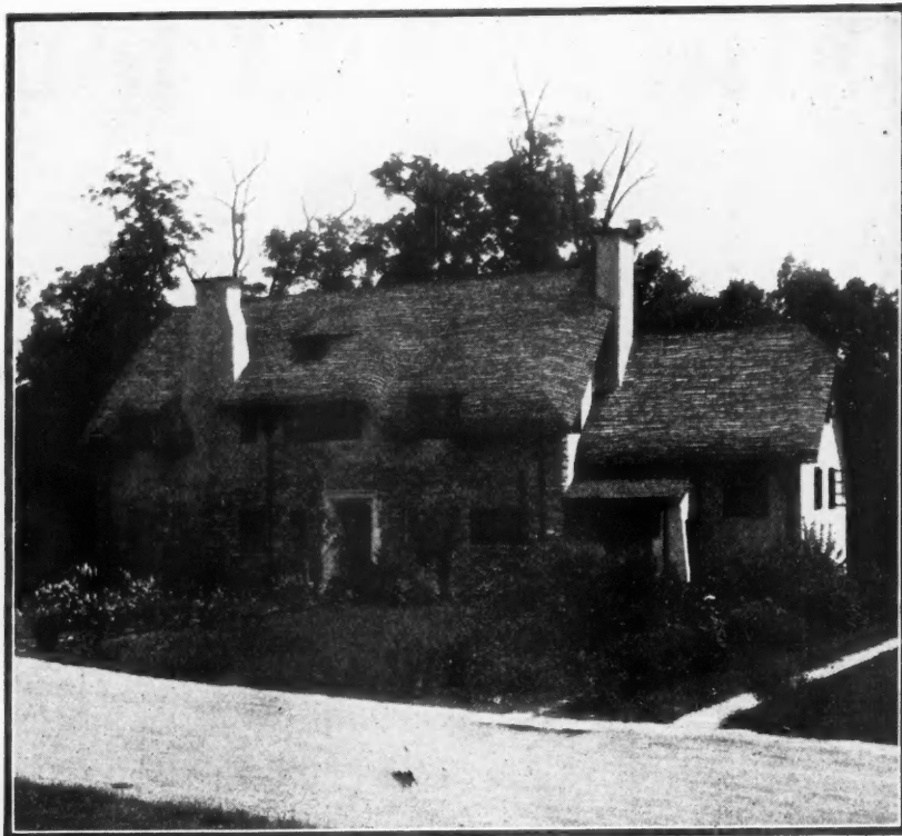
Res. of James Gilmore, Esq., Reg. Arch. Cincinnati, Ohio, Bishopric Ivoral Cream Stucco over Bishopric Base on all exteriors.
