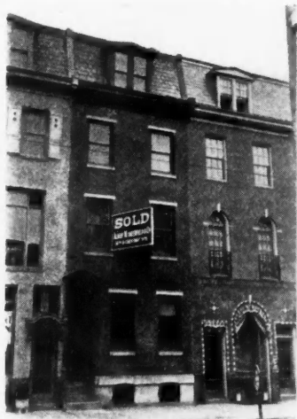
This Building at 221 South Seventh Street, Philadelphia, Had Little to Commend It Until It Was Given a New Front as Shown Below.
