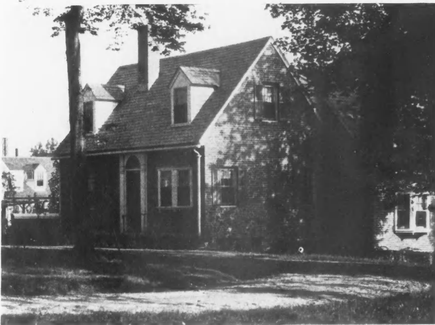
Bay Windows and Roof Dormers Were Standardized as to Size and Design, Then Built in the Shop, and Delivered to Each Job Complete, Ready for Installing.
