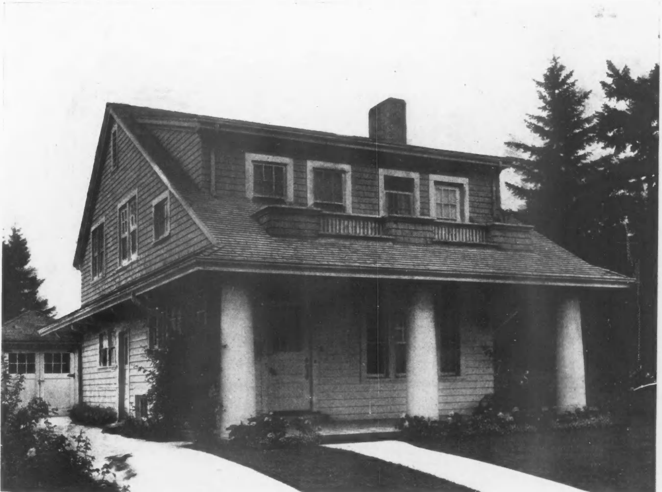
Photograph of Our Front Cover Home. Working drawings made to \frac{1}{8} -inch scale are presented on the four pages following.
