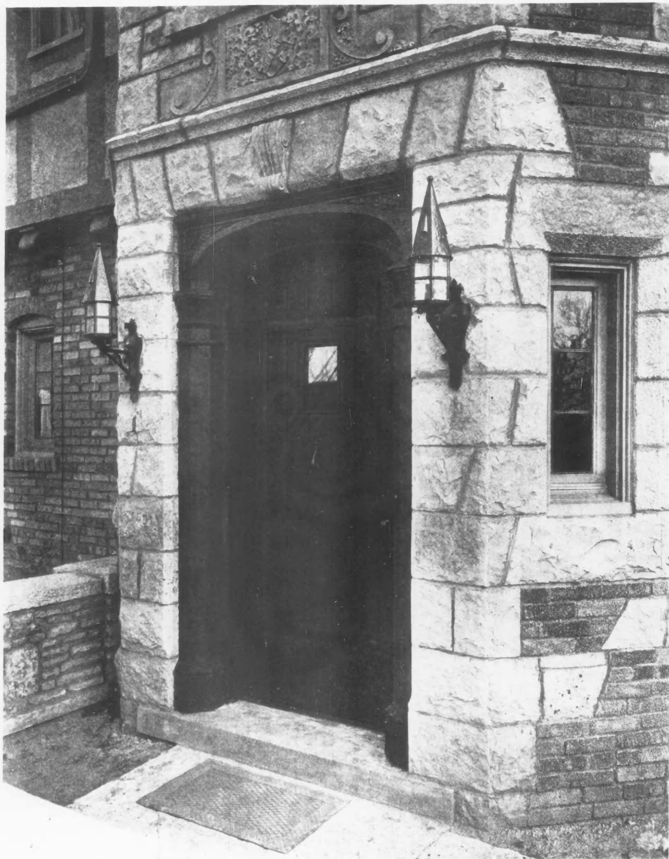
The Entrance to the New Home of Frank F. Hase, Well Known Manufacturer of Contractors' Equipment, Milwaukee, Wis., Features the Rough Hewn Timbers and Hand-Wrought Hardware, and Quaint Side Lanterns of an Earlier Day. The architect, Thomas Van Alyea, of Milwaukee, has handled these details in connection with the light gray brick walls and Lannon stone trim in a most commendable style. It is interesting that Dan Danielson, the contractor, using his regular equipment, mixed all the mortar for this house with a power mortar mixer, and ran all the millwork on a power saw rig, both of Mr. Hase's manufacture.
