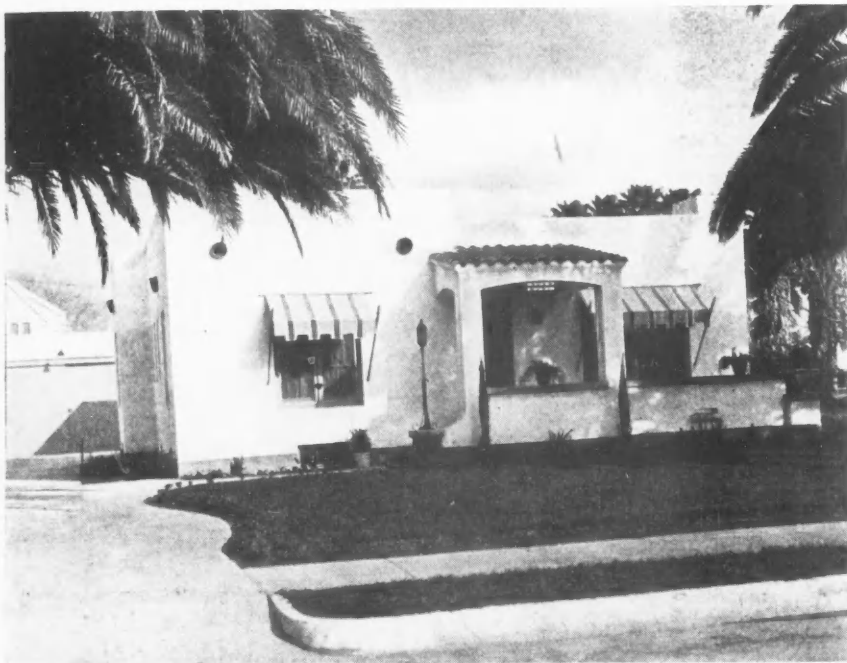
Photos and Floor Plan of Beautiful Spanish Bungalow Built by Contractor Fluor Near Los Angeles. An example of his reinforced concrete veneer.
