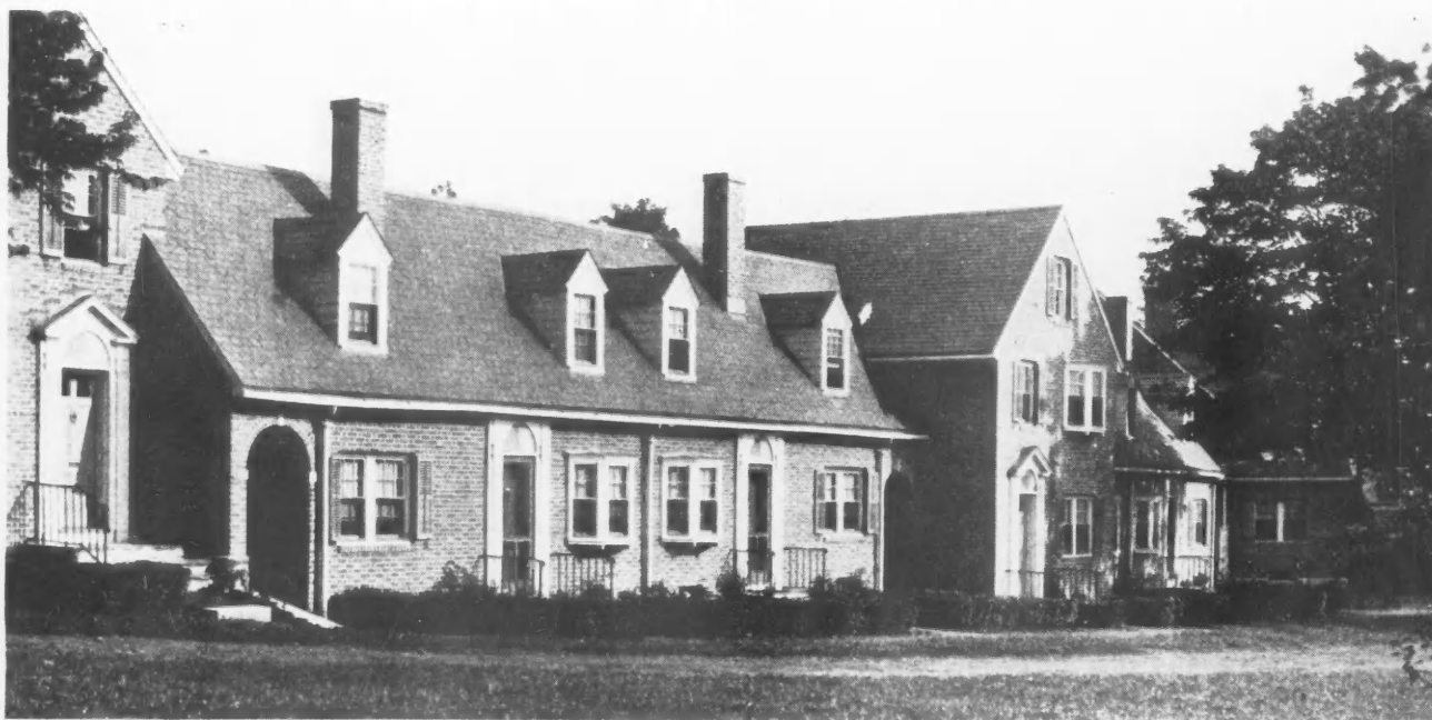
The Architects of Rippowam Village, Perry, Shaw & Hepburn, of New York, Used Great Skill in Combining Standardized Elements, Such as Colonial Entrances, Projecting Bay Windows and Roof Dormers, in Such a Way as to Give Variety and Picturesqueness to the Whole Group of Houses at Rippowam Village, at the Same Time Keeping the Cost to a Minimum.
