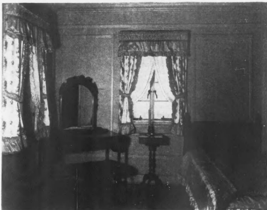
The Bedrooms in the Demonstration Home Are Tastefully Furnished. Notice the steel casement windows. The walls and ceiling are attractively panelled with sound deadening and insulating board.
