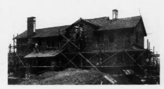
The Completed Rheinfrank Residence Is Shown Above While Just Below It Is Seen in the Course of Construction Showing the Tile Walls Construction.
