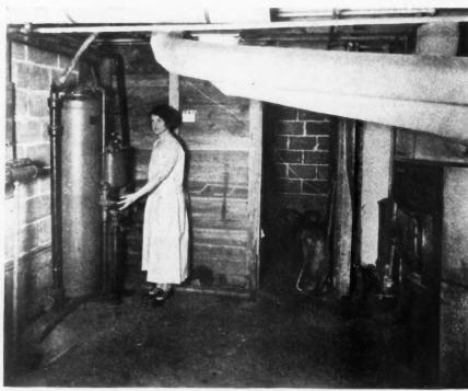
A Water Softener Occupies Only a Small Space in the Basement, but It Makes Available an Ample Supply of Clean, Soft Water at All Times and Costs Less Than a Cistern in the Long Run.
