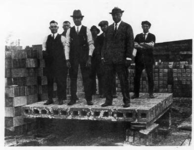
Eight by 8-Foot Straub Block Wall Laid Down; Supported Seven Men and Several Cinder Blocks Before Rupture. Note mortar joints—buttered on edges only.
