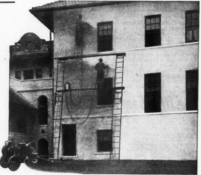
gives you all that is practical, complete and reliable in spray-painting equipment. The DeVilbiss spray gun operates on the lowest practicable air pressure; it makes possible 4 to 5 times faster painting than can be done with the hand brush; it insures a more thorough and uniform coating with any kind of paint, on any inside and outside surface.
