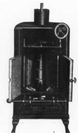
A Baffle Plate with Telescoping Support Forces the Refuses Down and Automatically Shuts Off the Gas.
