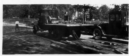
Fig. 2. Power for Moving the House Was Furnished by This Motor Truck Equipped with a Winch.
