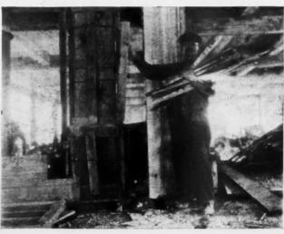
All Debris and Pieces of Wood Are Removed from the Floor by This Chute Passing Through a Light Well.
