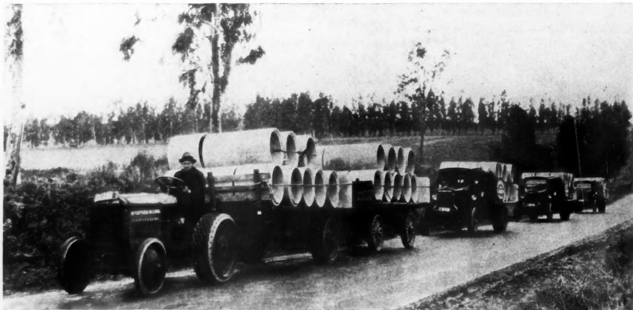
Two Methods of Handling Large Tile Which Have Proved Practical and Economical. For such loads as this, however, there is probably greater economy in the tractor-trailer unit in front than in the single truck loads behind, especially as there is probably no rush element involved in this delivery.
