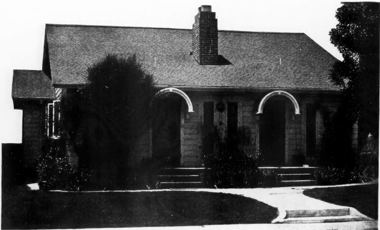
A Simple Frame Cottage Which Will Accommodate Two Families in Perfect Comfort and Privacy. The well-designed entrances, with their arched roofs, are tied together by the tall narrow windows, overcoming the duplex suggestion of the double entrance.
