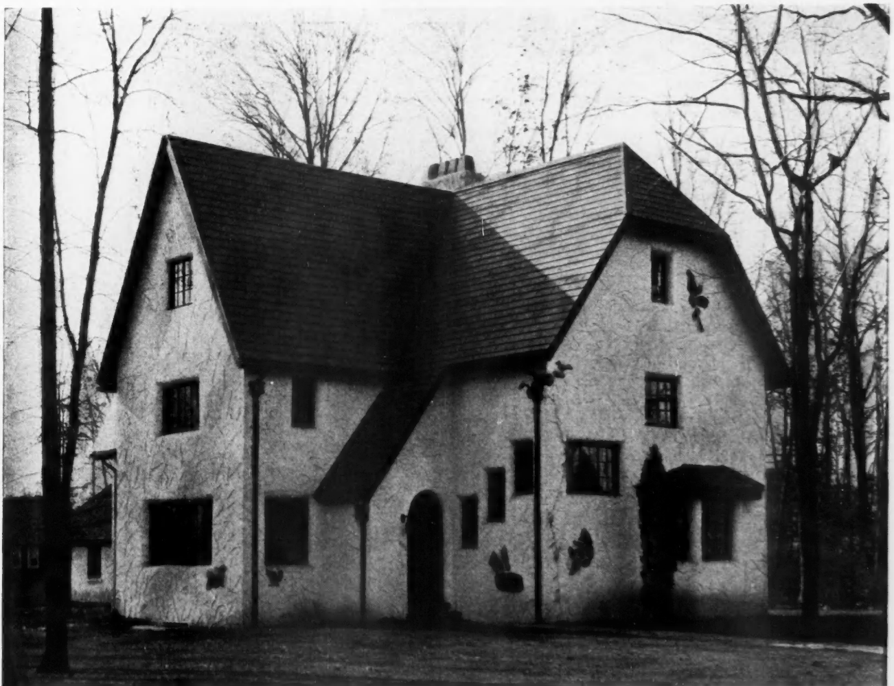
Mrs. Trimble's Home in Westfield, N. J., Built from Her Own Plans. It is attractive and comfortable within and without. The walls are of hollow tile with stucco which has been given a special rough texture.
