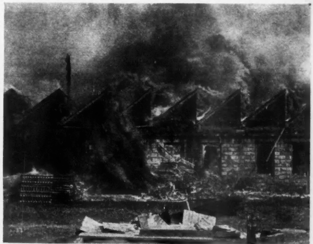
A Small Fire and a Strong Wind and the Roof Is Lost. So also may be the other surrounding buildings which are exposed to flying sparks.
