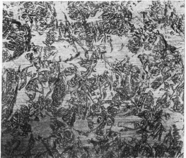
A Handsome New Wall Finish Achieved with Paint and a Special Spray Brush. The effect is pleasing and the wall has the added advantage of being washable.
