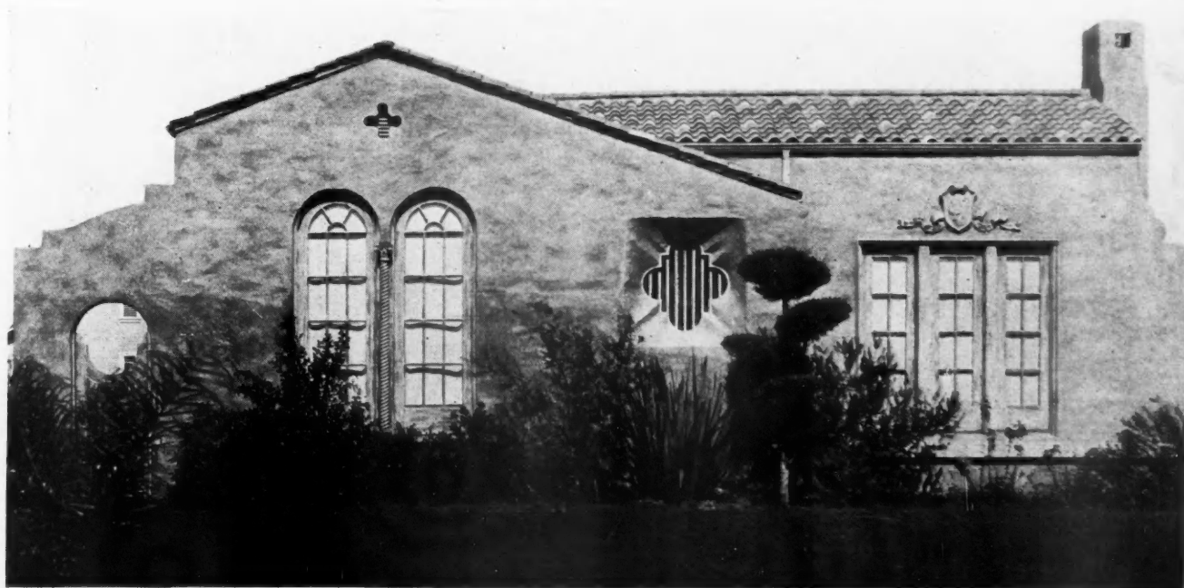
The Exterior of This Spanish Home Presents a Number of Distinctive Details. The stucco finish gives the effect of crinkled parchment, the vestibule window is most unusual in design and the design of the other windows is strikingly individual.
