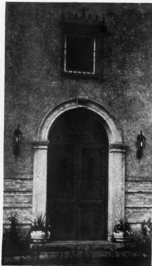
Paneled Oak Entrance Doors, Flanked by Wrought Iron Lamps, and the Wrought Iron Grill Over the Stair Window Above Are Touches Which Carry Out the Italian Tone of the Ritter Apartments, Denver, Colo.
