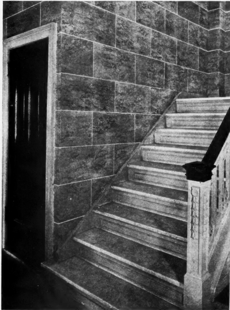
Under Conditions Where Ordinary Plaster Would Not Meet the Requirements, Keene's Cement Is Used. This includes such work as wainscote, finishing columns, and making Caen stone and Travertine finish.
