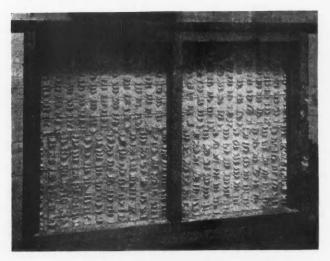
As the New Type of Lath Appears from Behind, Showing the Keying of the Plaster Through the Perforations.
