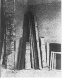
The Casing, Jamb and Head Moulding for Each Door Should Be Carefully Removed and Tied in One Bundle.
