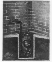
b. 382. Construction of "Pen-Berthy" Automatic Con-No. 382. DRAINER
