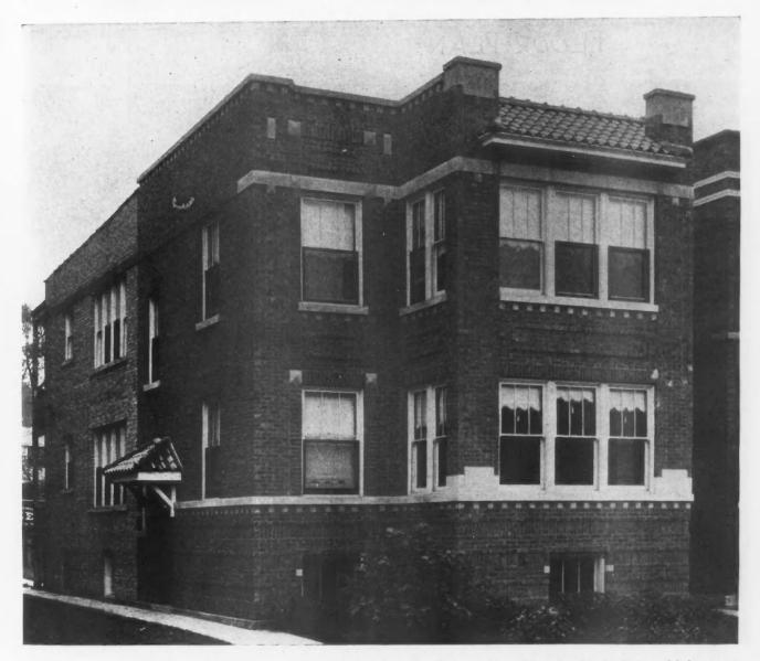
The Above Is an Excellent Design for a Two-Flat Building on a Narrow Lot. The wide bay in front, with its seven windows on each floor, is a desirable feature for light and air. The plan shows a conveniently arranged five-room suite on each floor and practically no waste hall space. The living room is commodious, 20 feet by 21 feet six inches, and has an unusual number of windows.
