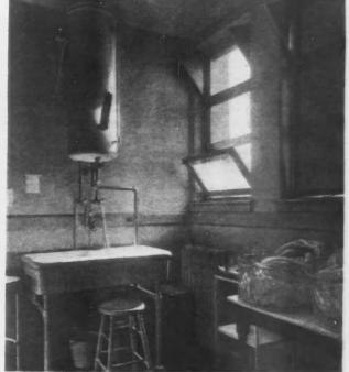
View of Baby Bath. Note the stall type of window which allows ventilation without direct draft.
