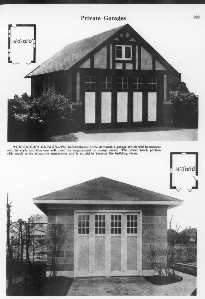
THE SAFFORD GARAGE—Concrete blocks can well be used in building the garage, especially when the house is of the same construction. It is as well adapted to the small single car garage as to the larger types. Its appearance is always good and has the quality of permanence in a high degree. AMERICAN BUILDER (Covers the Entire Building Field)
