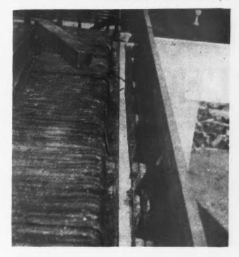
Forms in Position for Casting a Tin-Pan Type Floor. Note the beam reinforcing and the metal lath used over the air spaces in walls to prevent the concrete from entering the latter.
