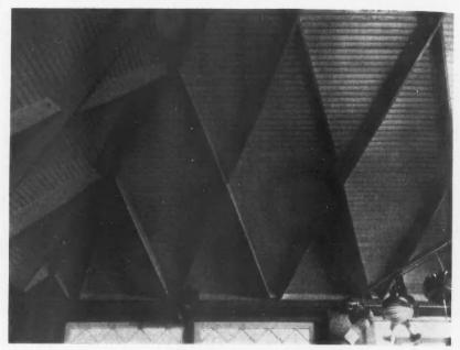
One Corner of a Large Exhibition Hall Gives a Clear Idea of the Appearance of this New Type of Roof Construction Which Has Recently Come to Us from Europe.
