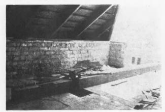
This Is Probably the Most Satisfactory Method of Holding the Timber for Supporting the Hoisting Pulley.
