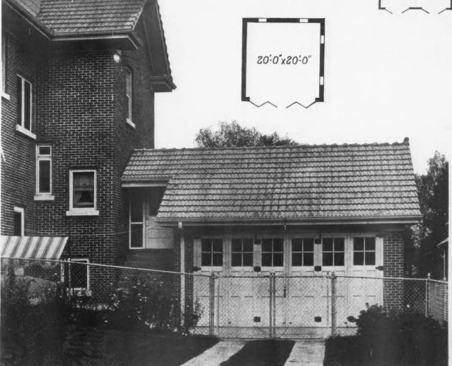
THE SECOR GARAGE—Not only does this garage follow the style of its house, but is attached to it with the appearance of being an actual part of the structure. It is, however, separated from the house structure by a solid wall, which is a requirement under the fire regulations of certain communities.
