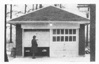
Doors Which Slide Up Into an Overhead Position Are Always Out of the Way, Are Never Damaged by Being Banged by the Wind and Are Not Injured by Rain, Snow or Ice.
