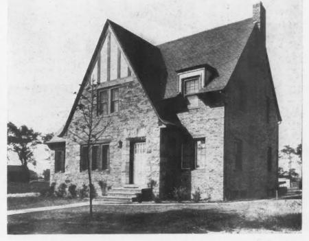
Where Hollow Brick Walls Are Used to Good Effect. Below grade the basement has 12-inch all-rolok walls while the first and second stories and gable ends have 8-inch rolok-bak walls.
