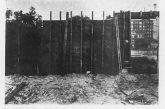
Sheathing Can Be Stripped from the Studs Without Damage by Knocking It Off with the Front of a Pick.
