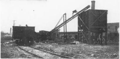
Elevated Aggregate Bins and Automatic Loader Make Possible the Efficiency of Gravity Feed Throughout the Plant. This view was taken at the plant of the Best Block Company, Milwaukee, Wis.
