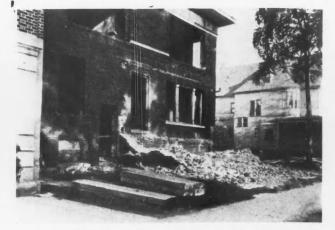
The Second Step Is to Remove All Projections. Here the front porch is being taken down and the cut stone copings carefully laid aside.
