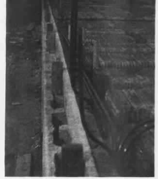
End Board and Floor Forms in Position for Casting the Beam and Arch Floor.
