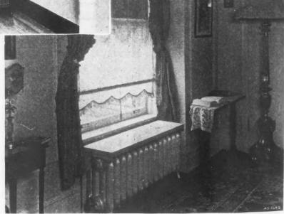
Radiator Furniture Not Only Improves the Appearance of the Room but Also Improves the Heating Efficiency as Well. A large quantity of water can be evaporated from the pan under the ornamental seat assuring healthful moisture in the home.
