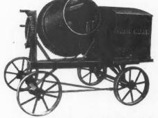
A Concrete Mixer of a Size Especially Adapted to General Construction, Foundation and Sidewalk Work in an Improved Model.
