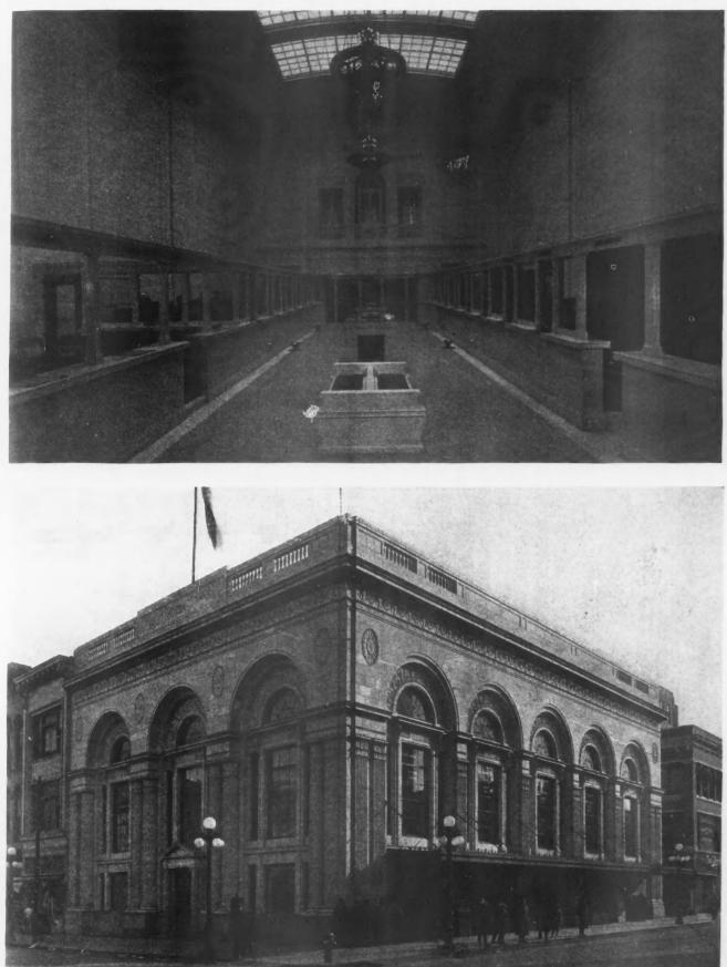
Kalamazoo Trust and Savings Bank Building, Kalamazoo, Mich., Weary and Alford, Chicago, Architects. The building is of reinforced concrete and has two large steel girders which span the banking room. An economic feature of this building is that space has been provided for a number of high class shops, and revenue from these leases is said to be sufficient to carry the investment in the entire building.
