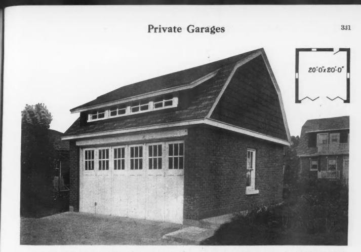
THE SAINT CLAIR GARAGE—Another attractive design, for the larger brick residence, is of brick and shingle construction with a composition shingle used on the roof. It is of a size to provide for housing of two cars and its plentiful lighting will be found a great convenience.
