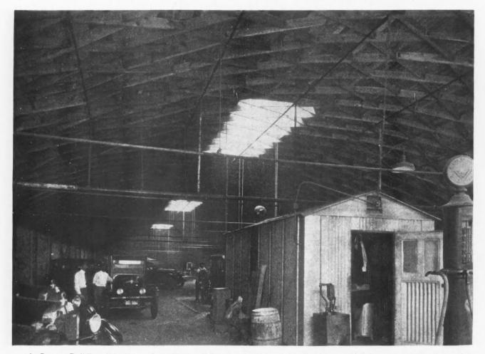
A Garage Building Where the Lamella Roof Construction Has Been Used to Good Advantage. This is the flat, segmental arch type with the thrust taken up by tie rods which can be seen suspended from the roof. The pipes shown in picture are sprinkler pipes.
