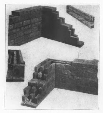
Fig. 3. The All-Rolok Wall Is Constructed with Two Courses of Brick on Edge Followed by a Flat Header Course. It is useful for stucco finish and for interior walls.
