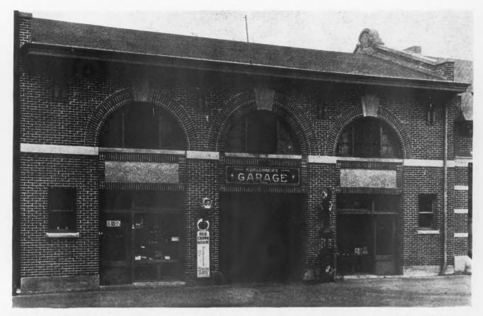
This Is a Well Designed Garage Building with Attractive Architectural Features. Piers are introduced in the brick walls to carry the roof trusses and to add stability to the 96-foot long walls. Three skylights light and ventilate the interior.
