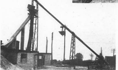
Bucket Conveyor and Gravity Chute Handling Aggregate at the Plant of the Steward-Silver Company, Columbus, Ohio. This method shows efficiency in some plants. View at the Delta Brick & Tile Company's Plant, Detroit, Mich., Showing Belt Conveyor in Use Bringing Concrete Blocks to the Storage Yard. ma oth
