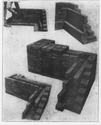
Fig. 2. The 12-Inch Standard Rolok-Bak Wall. The outer brick are laid flat and the back-up is of brick laid on edge.
