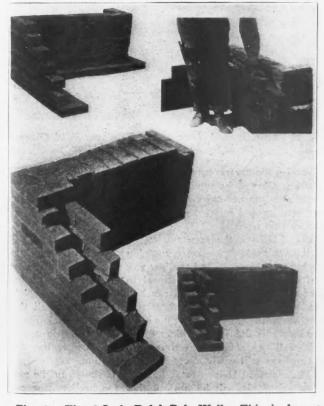
Fig. 1. The 8-Inch Rolok-Bak Wall. This is lowest cost type of hollow brick wall. It has the appearance of solid brick.
