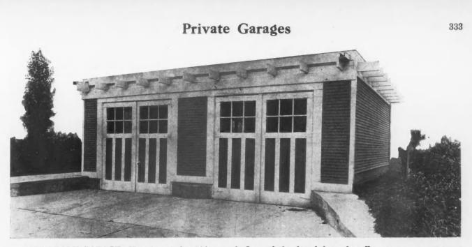
THE SEALY GARAGE—Here is a design with a nearly flat roof, the slope being only sufficient for draining, which has been given an added degree of individuality by projecting rafters which are suggestive of the pergola.
