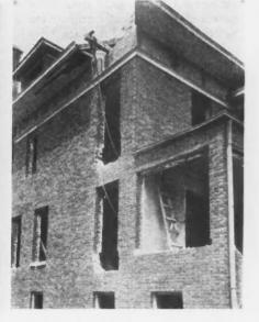
Pulleys Suspended from a Beam to Lower Steam Radiators, and Plumbing Fixtures to the Salvage Truck.
