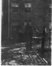
Here Is the Method of Taking Up Floors so as to Save the Material for Further Use.
