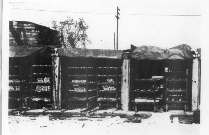
The Elimination of Waste Space in Curing Tunnels Makes a Direct Saving in the Amount of Steam Heat Required. These tunnels at the tile plant of the Superior Sand & Gravel Company, Detroit, Mich., are just long enough and high enough to admit the loaded cars.
