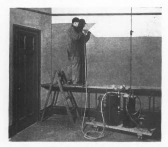
This Complete Unit for Applying Paint Lacquer, or Paint Remover, Is Mounted on a Truck on Four Casters, Making It Easily Portable.
