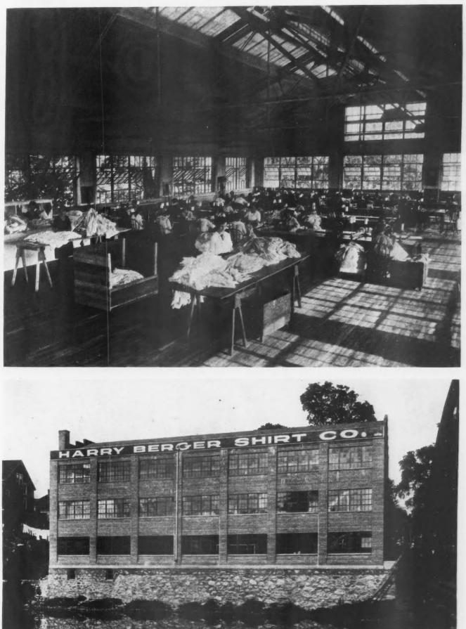
This Shirt Factory at Stamford, Conn., Provides Its Employees with Admirable Working Conditions, as Shown by the Interior Photograph. Note the clear floor space unimpeded by columns, due to the steel roof trusses, and the excellent light and ventilation provided by skylights and ventilating sash.
