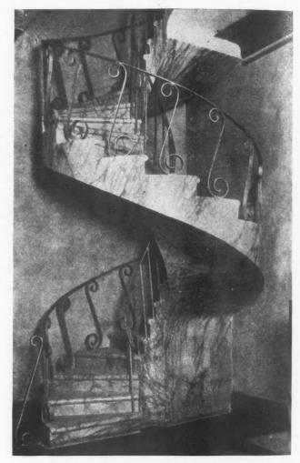
Probably the Only Existing Reinforced Concrete Staircase Without a Central Core Is Designed on the Principle of Perpendicular Balance.
