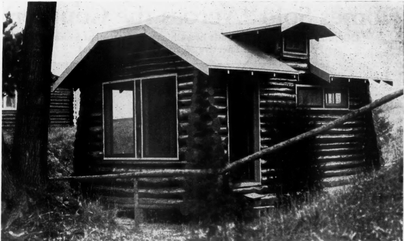
Even a Tiny House Like This May Be Made Attractive and Provide a Summer Cottage Which Offers a Plenty of Comfort and a Distinctive Charm. The cost of log construction is less than for frame construction from the same plans, and when properly built the log house is one of the most comfortable and satisfactory types of dwelling that has ever been devised.
