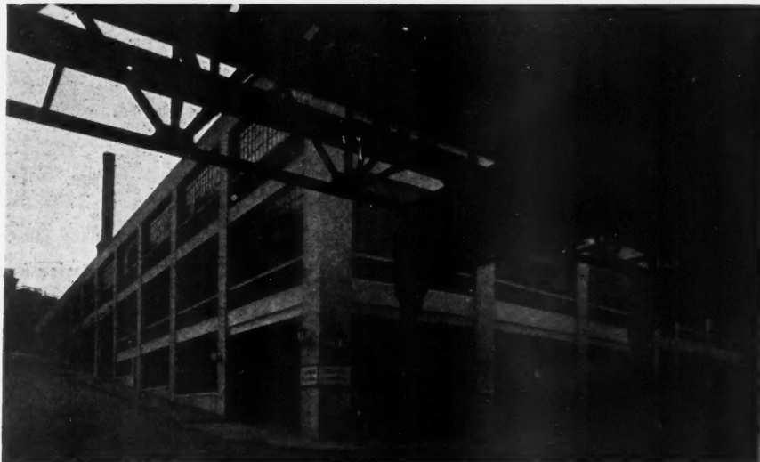
Only a View from the Air Would Reveal the Great Size of This New Truck Garage Which Accommodates Many Large Fleets of Trucks. No ramps or elevators are required as the sloping site allows entrance at grade to all three floors.
