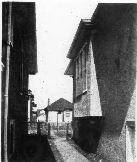
Fig. 2. A Small Bungalow Showing Good Construction in the Offset of the Eaves at the Bay Window.
