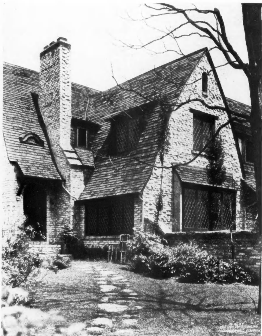
Skintled Brickwork, the Most Recent Step in the Development of New and Attractive Brick Walls, Originated Among Chicago Architects About Four Years Ago. This house is an example of the work of S. S. Bemen, architect.
