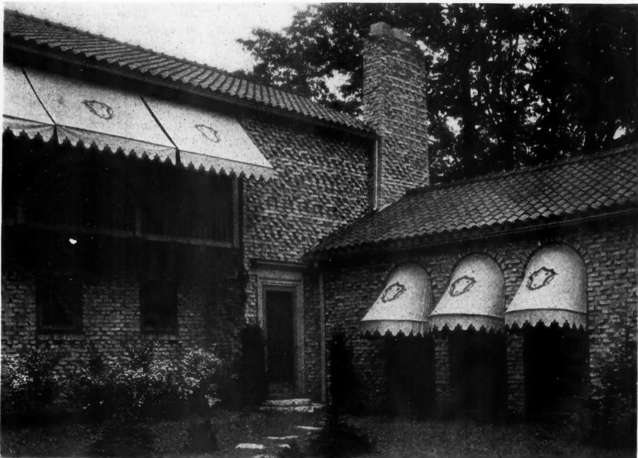
A Close-Up View of Skintled Brickwork as Used for a Home in One of the Fine Residential Suburbs Near Chicago, Showing the Beautiful Soft Texture of the Wall. James Roy Allen, architect.
