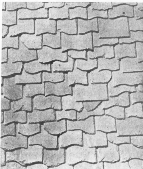
Section of a Thatched-Slate Roof
