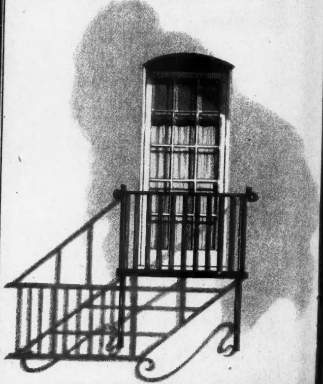
Detail of Wrought Iron Balcony for Full Length Window in the Large Front Bedroom.
