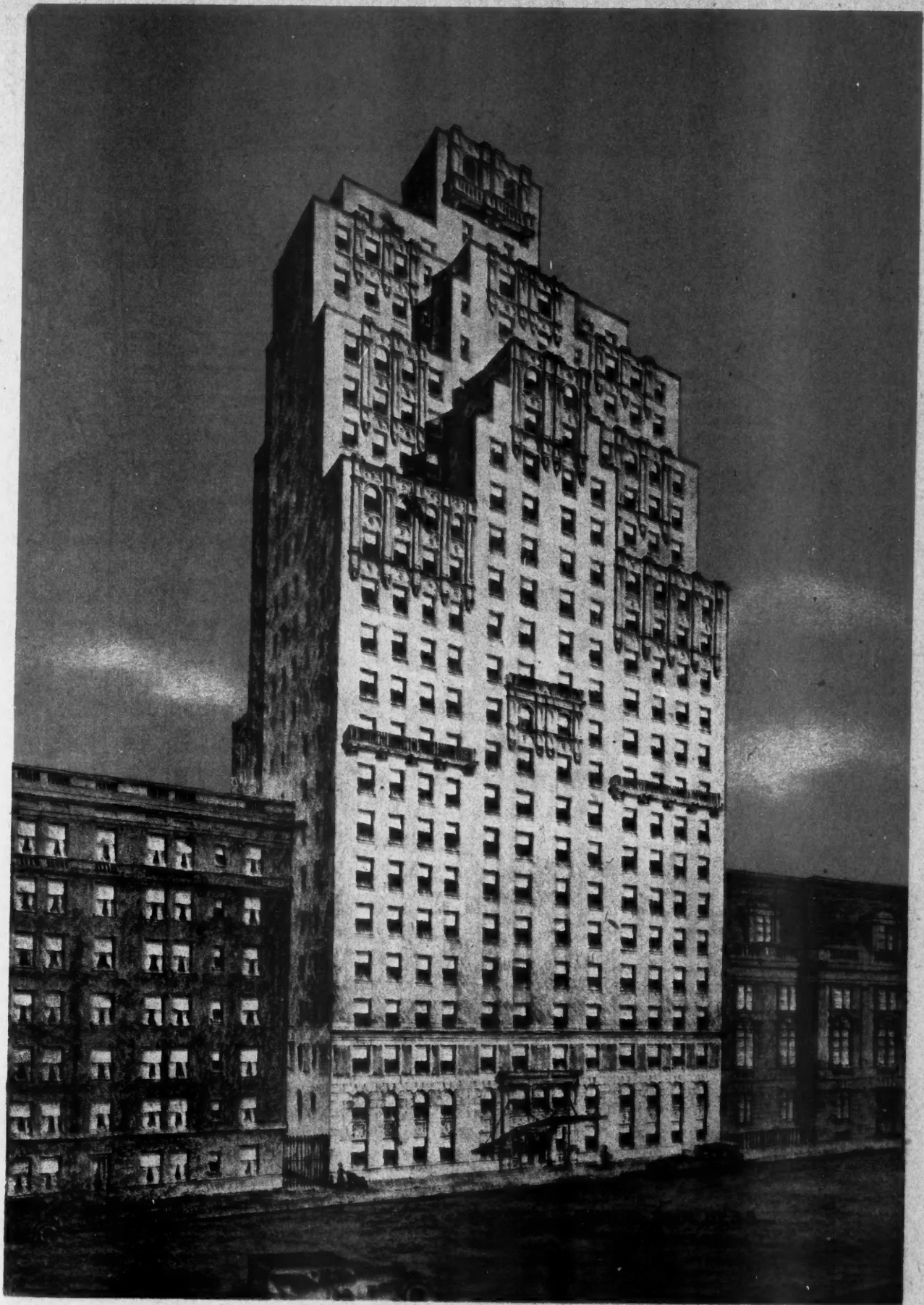
NEW APARTMENT HOTEL at 10 East 86th St., New York City; Arthur Paul Hess, of New York, Architect.
