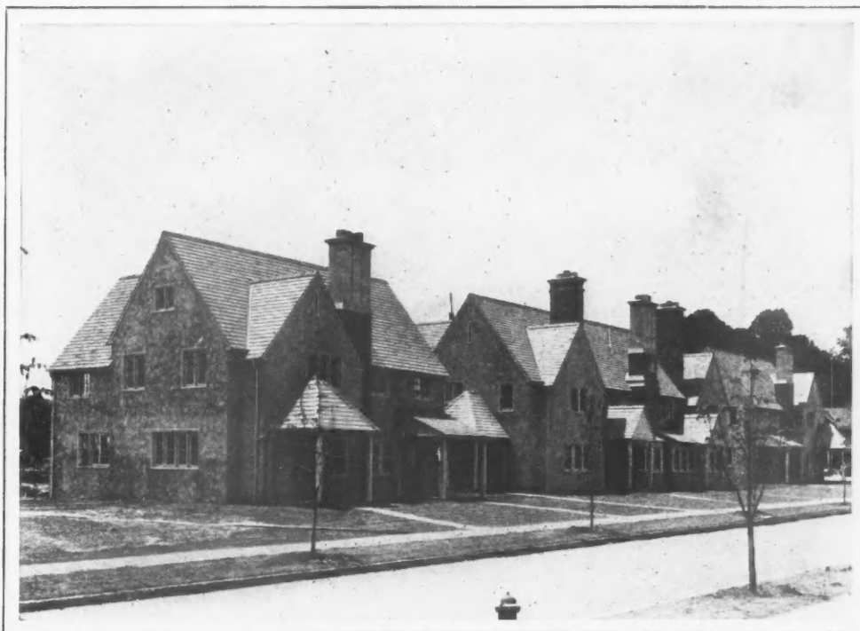
"Group" houses in Mariemont, near Cincinnati, Ohio; Carl A. Ziegler, Philadelphia, Architect. Kohler Plumbing Fixtures, extensively used throughout Mariemont, supplied by Walworth Co. and Mutual Mfg. & Supply Co., Cincinnati, Jobbers; installed by Ruhlman Plumbing Co., Mariemont
