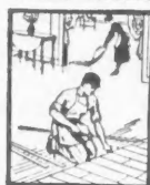
laid and used the same day
