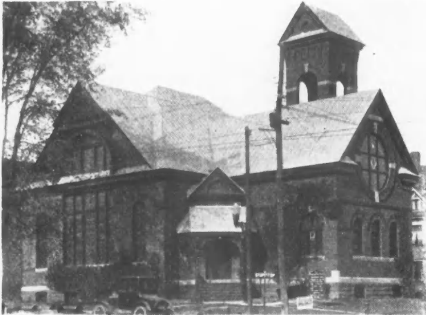
The First Congregational Church, of Fulton, N. Y., Is Roofed with a Permanent Roof of the Zinc Described Here.
