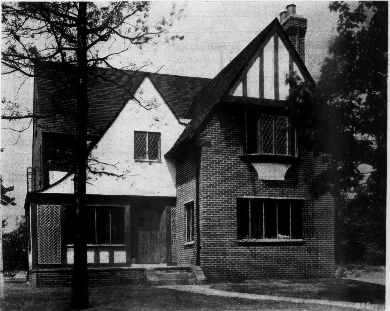
An English Type of House, with Solid Brick Walls, Rough Hewn Timbering in Stucco and Small Paned, Casement Windows, Is the Distinctive Piece of Architecture Which Is Illustrated, in Colors, on Page 1, as Our Front Cover Home. Complete plans are to be found on the following pages.
