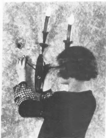
Attaching a Removable Light Fixture to the Convenience Outlet Which Gives a Double Purpose Outlet.
