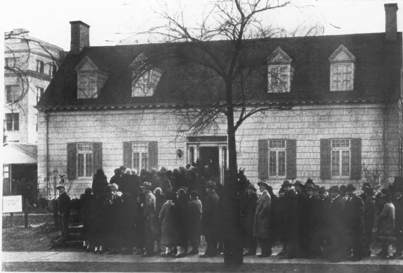
This Photo of a Demonstration Home Promoted and Built Under the Direction of Mr. L. Porter Moore and the Home Owners' Service Institute, Shows the Popular Interest That These Homes Always Create. Millions of home buyers and builders and their professional advisers will see, study and be influenced by these 36 "model" home demonstrations this year.
