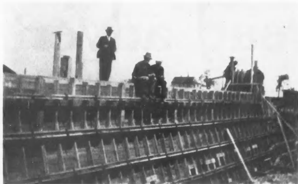
Using Form Clamps Which Eliminate All Wires and Permit Perfect Alignment of Forms by a Most Simple Means.
