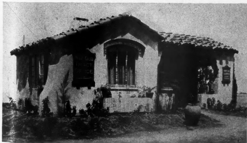
The Pacific Building Company Has So Designed This Attractive Spanish Style Office That It May Be Hoisted on Screw-jacks and Moved To a New Location When Business Demands.
