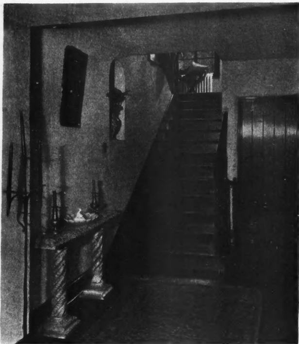
Fig. 12. A Curved Top Wall Niche, as in Figure 10, as It Appears When Finished.
