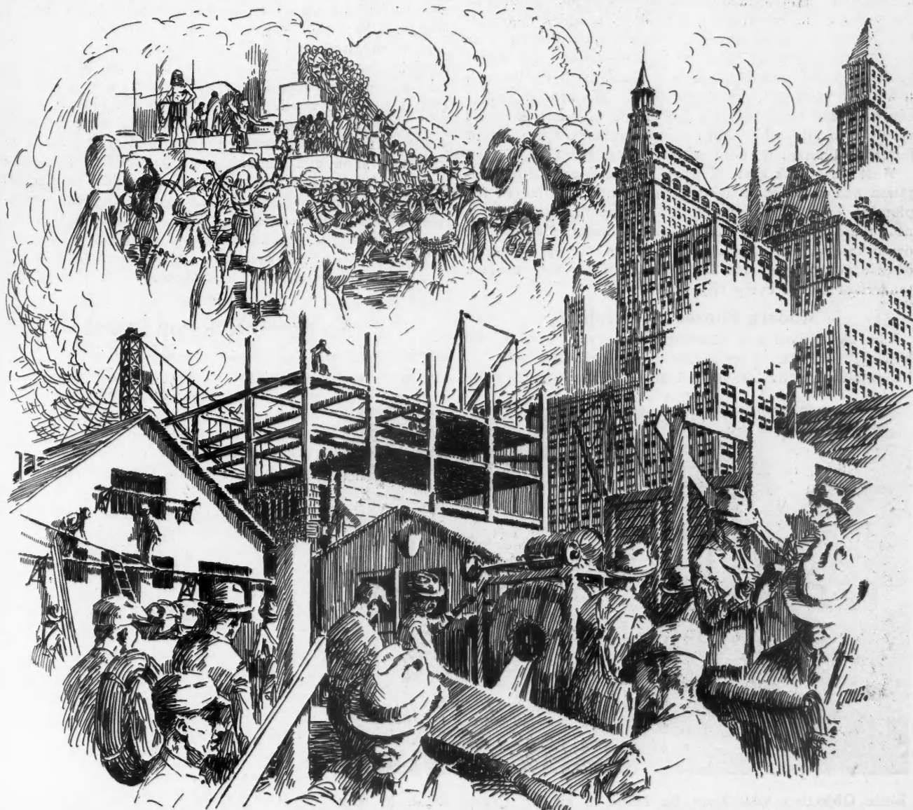
The Builder's Life Is Full of Romance. No Two Hours' Work in a Day Are Similar.
