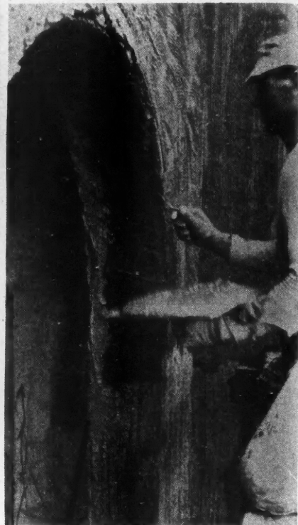
Fig. 11. Plastering an Arched Opening.
