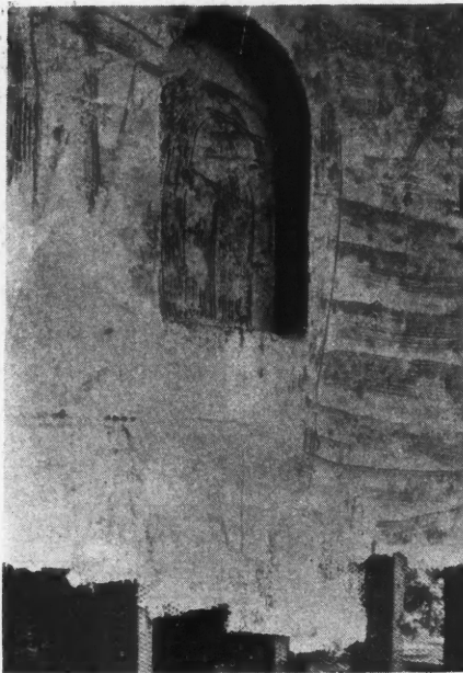
Fig. 10. Construction of a Curved Top Wall Niche for a Vase.
