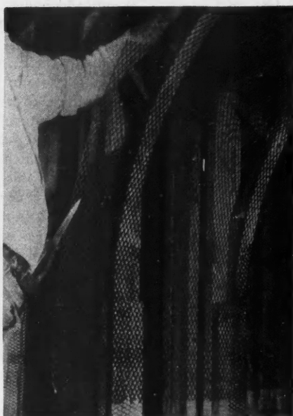
Fig. 6. Application of Metal Lath to an Arched Opening.
