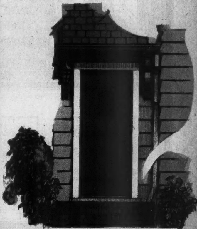
Detail of Quaint Entrance with Antique Hand-Forged Hardware.
