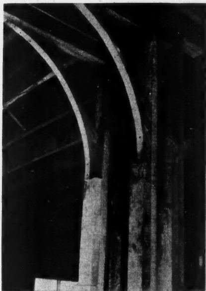
Fig. 5. Construction Detail for an Arched Opening.
