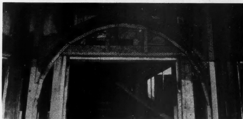
Fig. 8. Arch Construction Over the Flat Topped Doorway Shown in Fig. 4.
