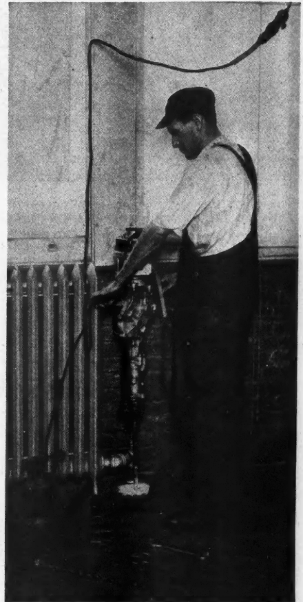
For Drilling All Kinds of Masonry This Pneumatic Drill Enables Rapid, Economical Work.
