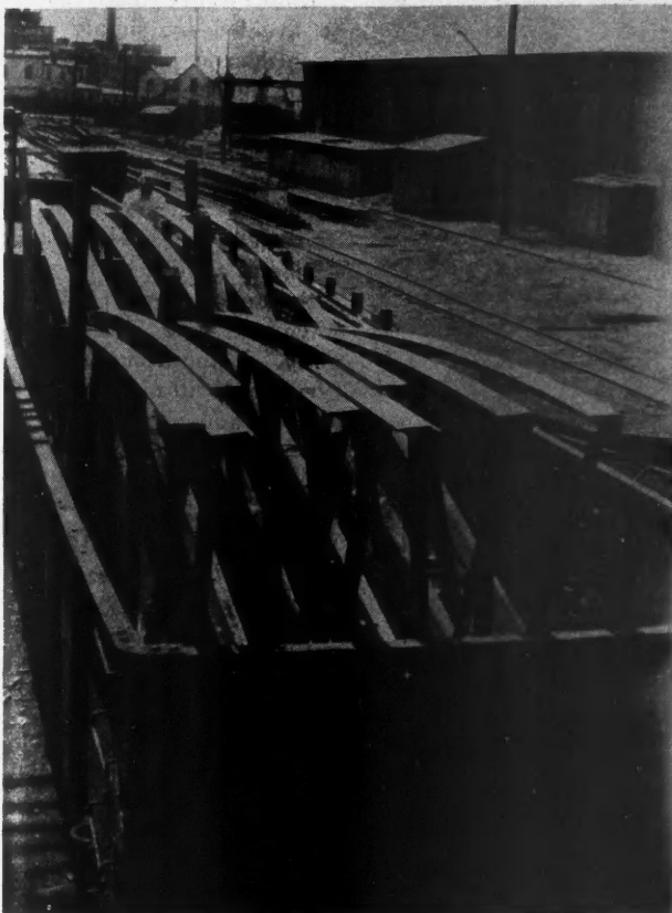
These Trusses Are Designed to Withstand, Without Damage, the Rough Handling of Shipment by Train, Boat or Truck.
