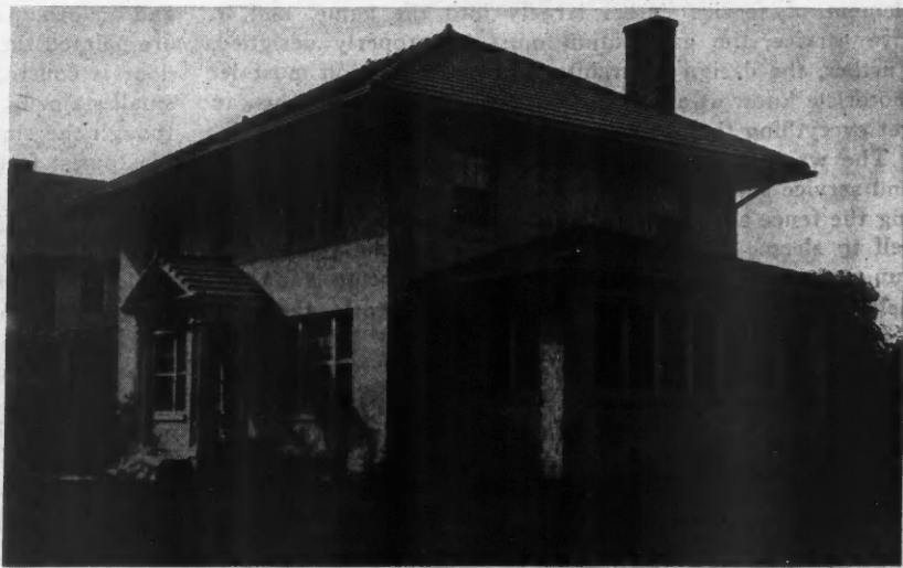
Permanence of Construction and Insulation Against Heat and Cold Were Demanded by the Owner of This House and the Methods Employed Have Given Complete Satisfaction.
