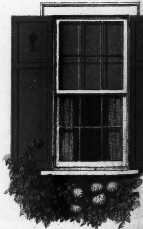
Detail of Colonial Window with Ornamental Shutters.
