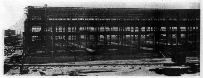
American Construction Methods, as Exemplified by the H. K. Ferguson Company, Are Finding Favor Among the Japanese, Where Rebuilding After the Earthquake Is Under Way. The illustration shows part of the \$10,000,000 plant the Ferguson Company is erecting for the Shibaure Engineering Works at Tsurumi, Japan.
