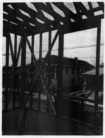
Note the Rafters Spiked to the Sides of Ceiling Joists in the Hurricane-Proof House. Also note the rafter heel plates on top of the ceiling joists, typical framing around the window, X-bracing in corners, herringbone bridging filling and open slots in the subfloor. The contractor carries proper public liability insurance during the demonstration period as protection against the possible injury of visitors.
