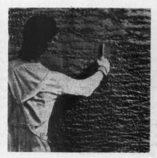
5. The Surface Is Then Worked Over with a Float.
