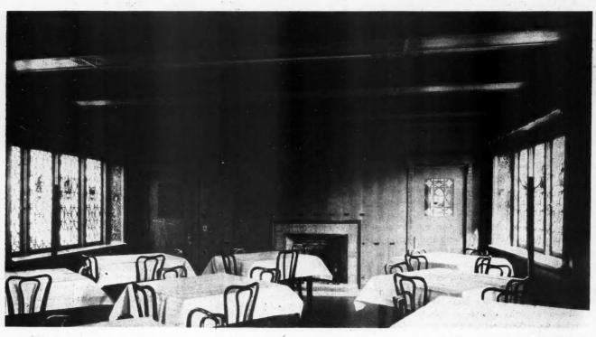
This View of the Men's Grill in the Emerson Hotel, Hoquiam, Washington, Shows How Fir Doors, Door Casings, Ceiling Beams and Recessed Panels All Received the Sand Blast Treatment Which Results in Such Uniquely Beautiful Effects at a Remarkably Low Cost.
