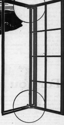
Notice how this friction control at both top and bottom of a Thorn casement holds the leaf open firmly at any position
