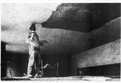
Applying the Brown Coat of Acoustical Plaster Over Half-Green and Scratched Base Coat of Gypsum Plaster. The application of this plaster is practically the same as that of ordinary plasters.
