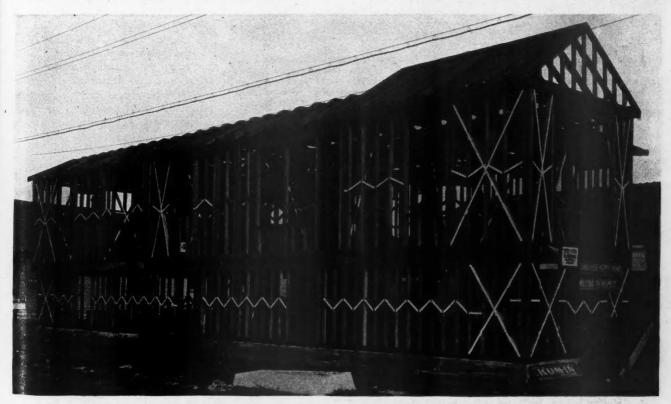
A General Exterior View of the Framework of the Hurricane-Proof House. The braces have been given one coat of paint to be seen plainly. The numbered signs on the frame correspond with the 15 points of good construction. There are two sets of these numbers scattered throughout the framework for the guidance of the public.
