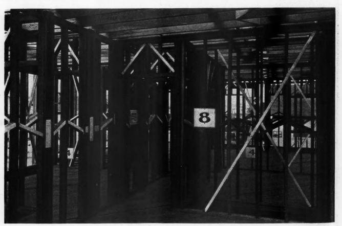
General Interior View. The thickly clustered study usually indicate where a partition or wall joins another, forming a vertical slot into which the walls, or partitions, fit and are blocked and spiked into position. Tying of walls to partitions and partitions to one another, is one of the urgent requirements for safety under powerful hammering and twisting storm stress.
