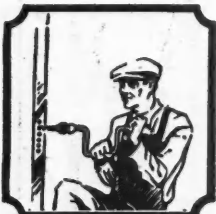
Only two mortises an hour this way.
