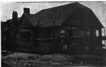
Douglas Fir sheathing, window and door frames, scaffolding, ladders and trim. The roof is covered with Western Red Cedar Shingles over Douglas Fir roofers. This house is built to last.
