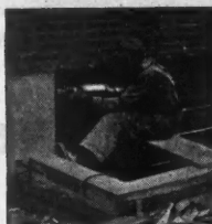
Bushing rough concrete surface
