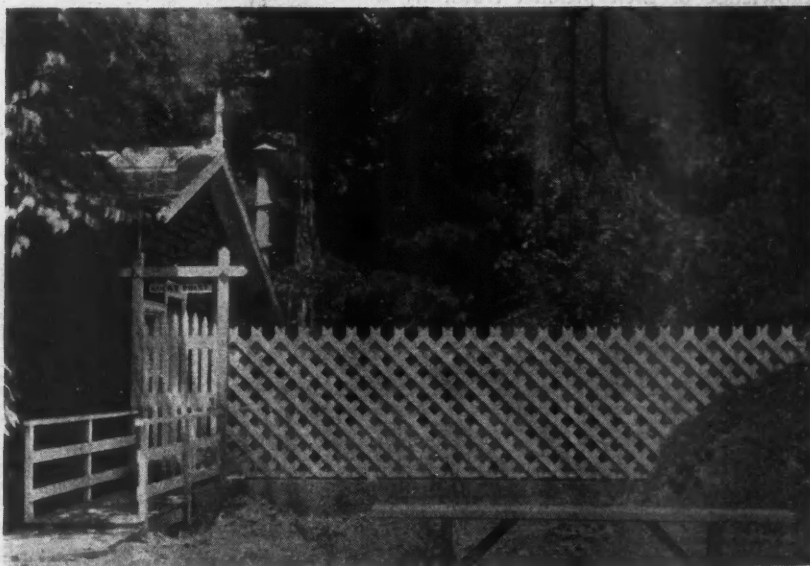
This Fence Was Built by Frank De Guerre, of Rocky Point, Villa Grande, California, from His Own, Original Design. It is inexpensive, quickly built and is described as "horse-high, cow-strong and pig-tight."
