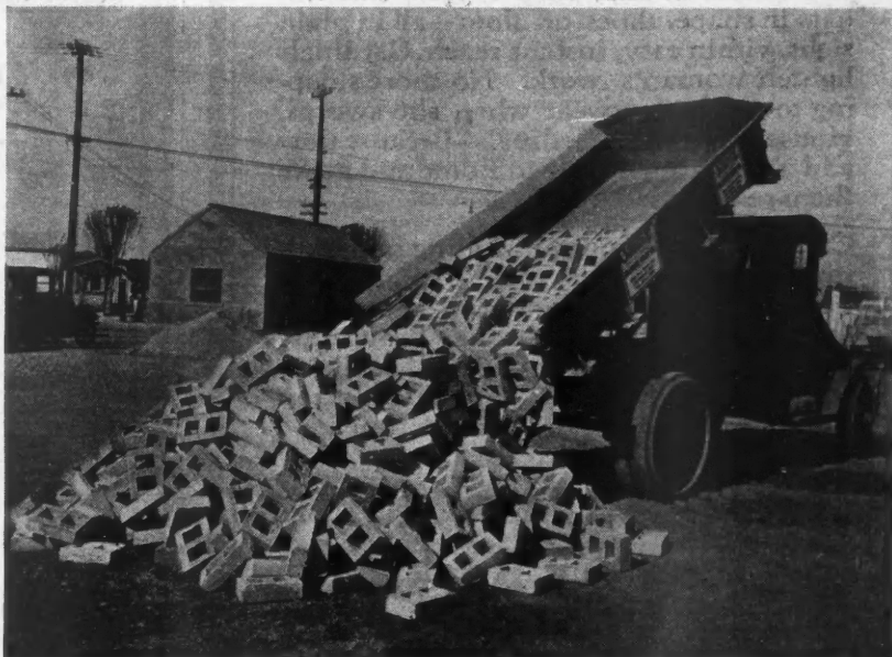
Unloading the Fillmore-Wiley Product Is a Quick and Simple Operation, Entirely Without the Breakage Which Accompanies the Dumping of Brick and Many Kinds of Building Block.
