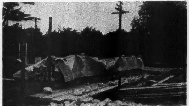
This Building Paper Is so Tough That After Being Used to Protect the Foundation It Was Still in Condition for Use in Sheathing.
