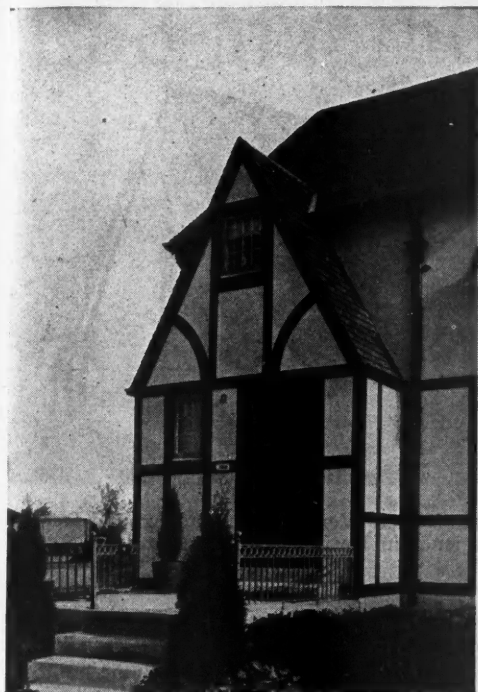
Entrance Detail of the W. A. Kuenzel Home, Which Was Built from the Plans of the Detroit Model Home.
