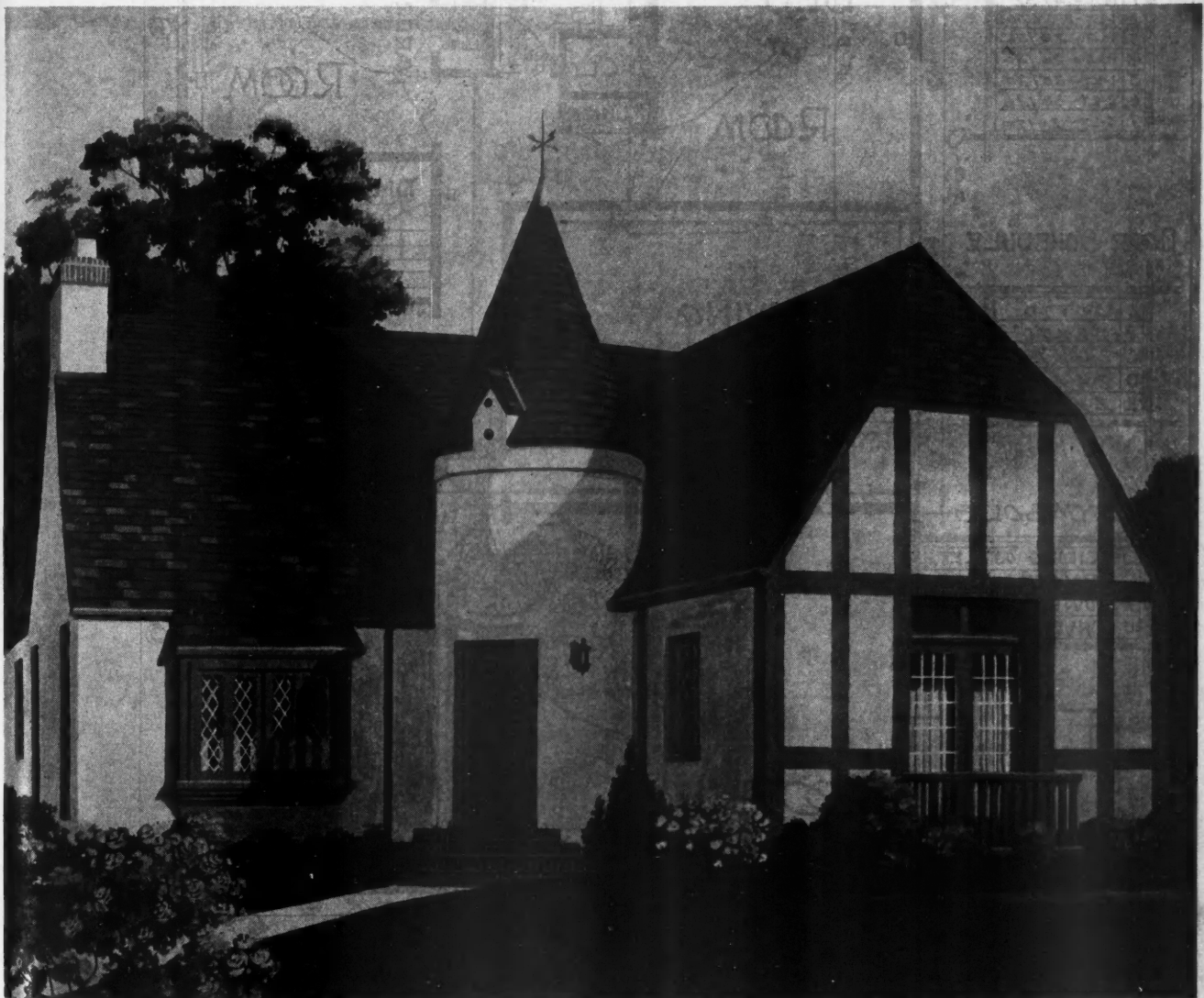
Norman Cottage of Five Rooms, Bath and Breakfast Alcove and with High Vaulted Ceilings in Dining Room, Living Room and Reception Hall. See the four pages following for complete working plans.
