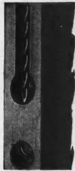
Two-hole sash. Drop chain through bore, slip hook onto end link and pull tight into bottom hole.
