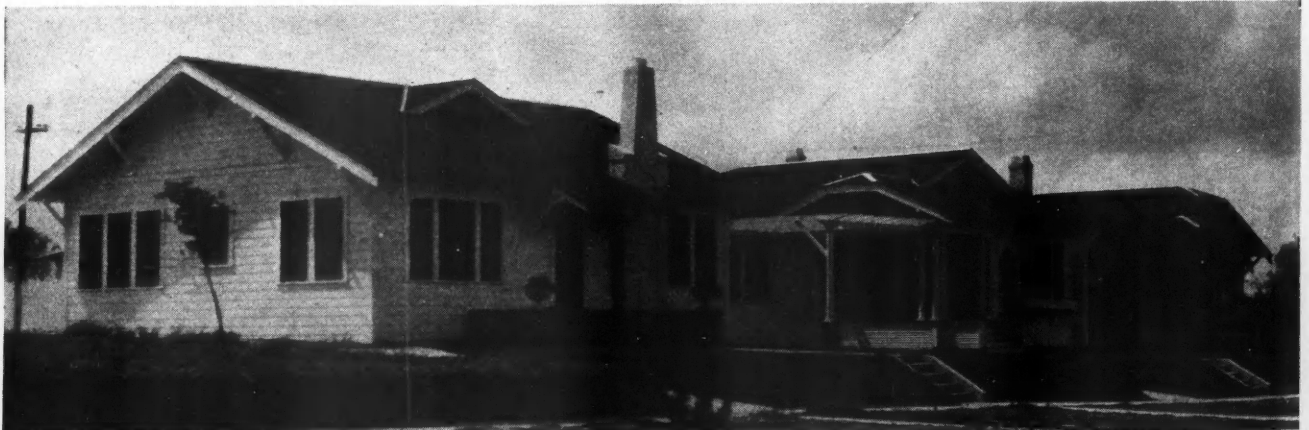
A Group of Homes Built by Mr. Klaus for Owners Who Had Already Bought and Were Thus Saved Interest Charges and Also Had an Opportunity to Put Their Own Ideas Into the Designs Made Especially for Them.
