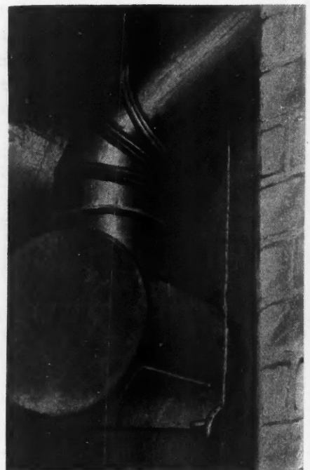
Smoke Pipes Made of a New Rust Resistant Metal Sheet Are Guaranteed for 10 Years Against Corrosion.
