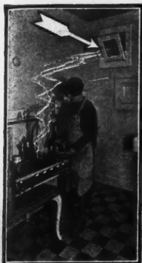
An ILGAIR Installation in an Oak Park, Illinois home. Note how the cooking odors, steam and fumes are removed.
