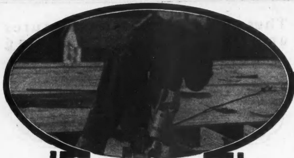
Cutting off Floor Joists or Sleepers
