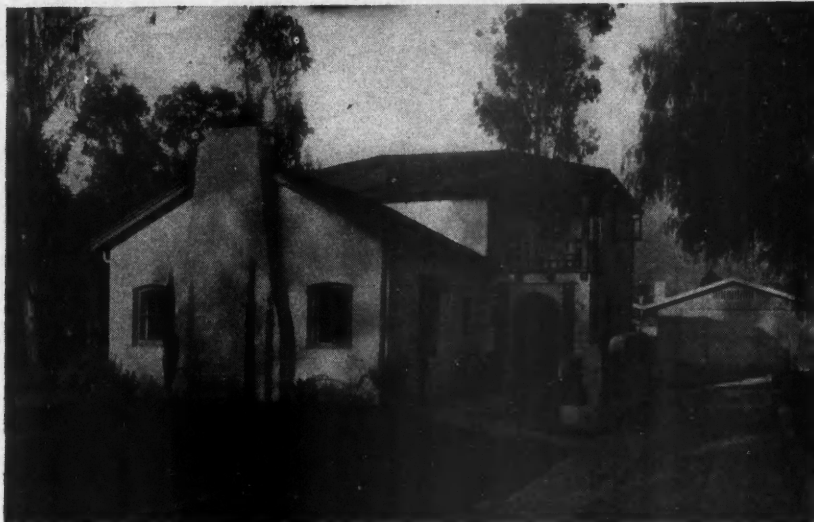
The Residence of F. C. Brittan, Jr., of Pasadena, Calif., Is One of a Large Number of Attractive Homes in That Los Angeles Suburb Built Entirely of the Fillmore-Wiley Tile.
