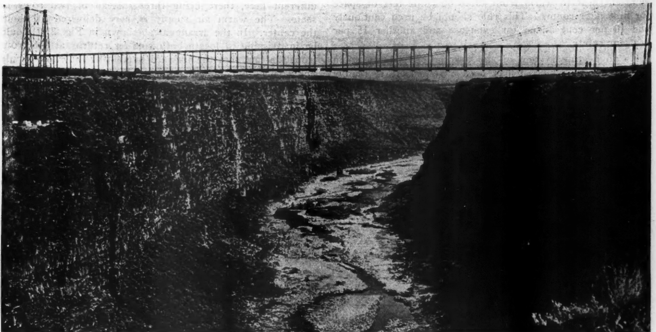
Six Hundred Ninety-nine Feet Long and 345 Feet High Is This Hansen Suspension Bridge Over the Snake River Near Hansen, Idaho.
