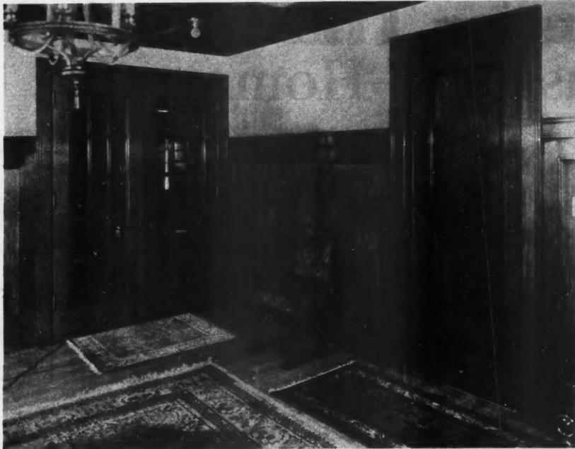
A Dining Room with Paneled Walls, the Panels Being Faced with Matched Veneers Taken from a Single Flitch, Is Particularly Pleasing.
