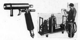
Here Is a Type of Spray Gun Which Is Said to Mark a Distinct Improvement When Used with This Company's Compressed Air Painting Outfit.
