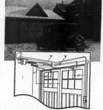
A Button Placed in a Post by the Driveway or Inside the House Opens and Closes the Garage Door.
