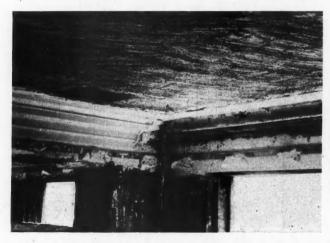
Fig. 3. The Portion of the Cornice at the Right Is Seen as Produced by the Rough Template While That at at Left Is Finished.
