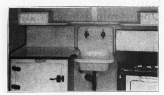
This Specialty Designed for the Small Kitchen of the Modern Apartment Combines Work Table and Drain Board, Fitting Over the Refrigerator.
