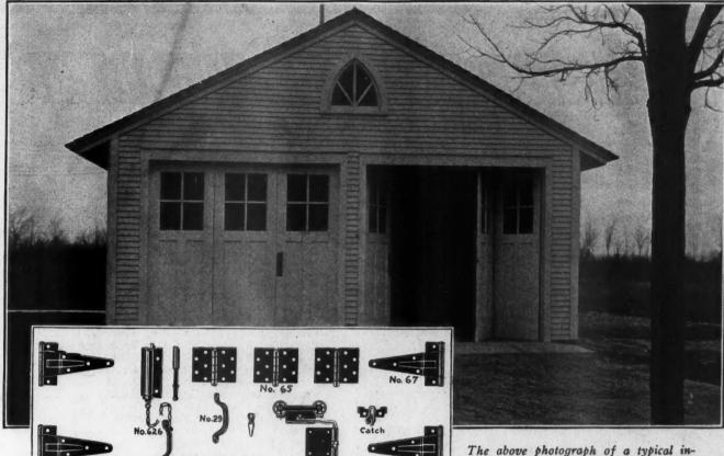
The above photograph of a typical installation of Frantz No. 50 "E-Z" Garage Door Fixtures shows how the doors fold neatly and easily out of the way. To the left are the items that make up this popular set.
