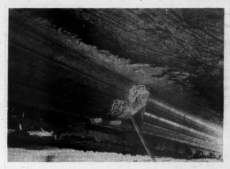
Fig. 5. The Finishing Template as It Appears in Use.
