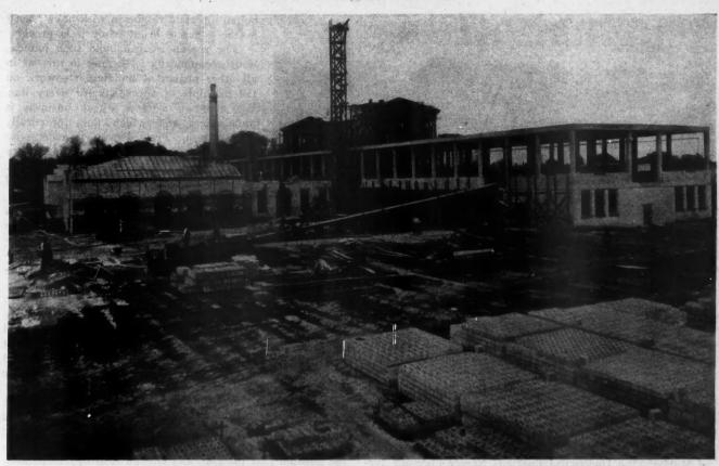
To Avoid the Expense of Shipping, a Concrete Block Plant Was Erected on the Site of the New Mobile High School and Here More Than 300,000 Tile Were Produced for Use in Its Construction. A separate tile company was organized for the production of the tile for this building.
