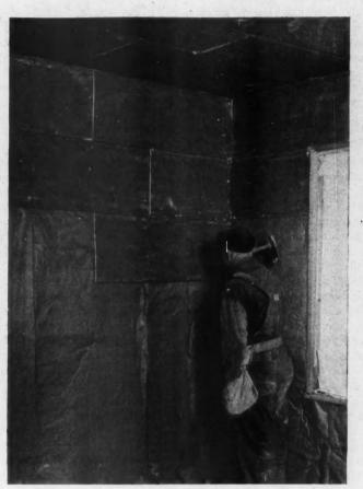
A Lather at Work in One of Mills and Sons' Westwood Houses. The photograph shows the insulation which is being used in the walls and ceiling and the application of gypsum lath, construction methods which play their part in producing first class houses.
