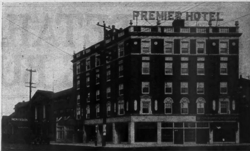
The Mineral Baths of the Premier Hotel, Benton Harbor, Are Lined with Mat Faced Tile Which Has Perfectly Withstood the Effects of the Minerals.
