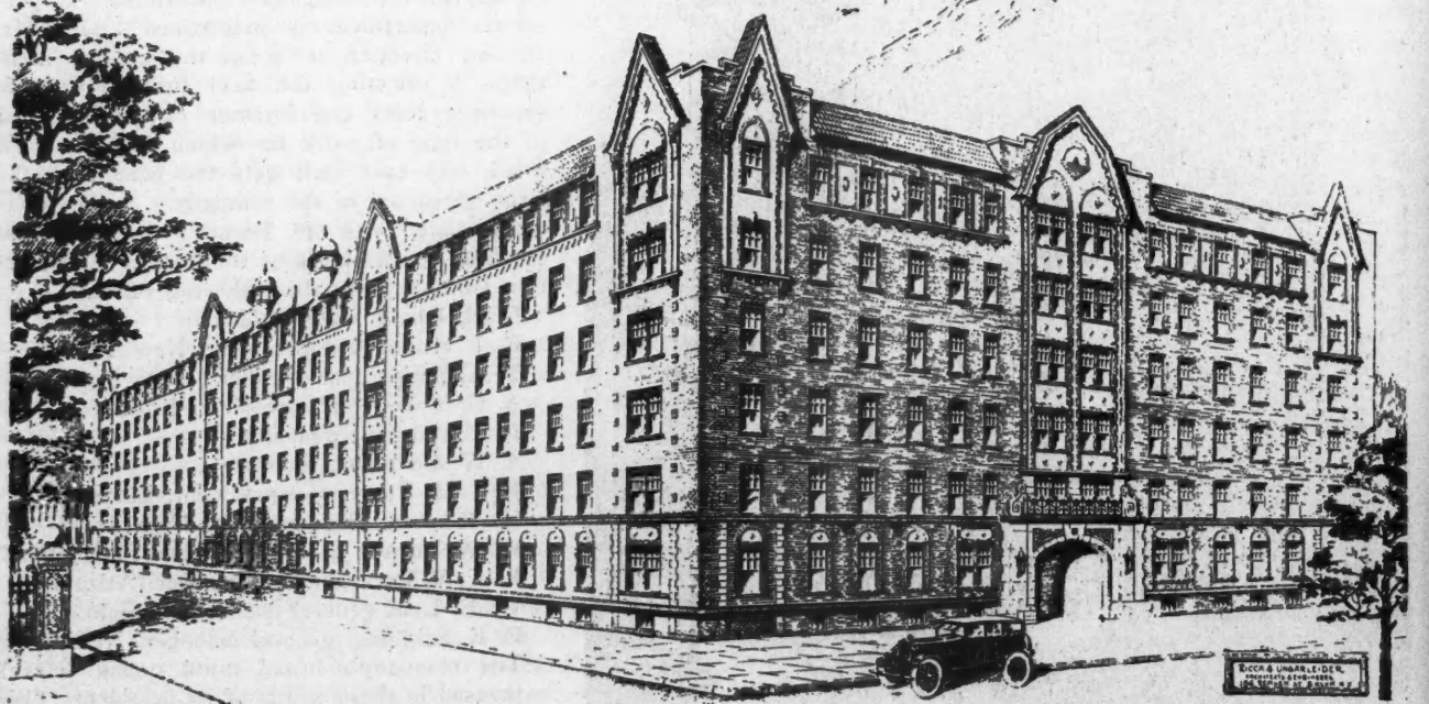
Tudor Elevations and Old English Half Timbering with Yellow Stucco Relieve the Mass of This Large Apartment Building Now Under Construction in Brooklyn. It is to be known as 1628 to 1640 Ocean Parkway, Brooklyn. Owners and builders are The Estate Road Building Corporation, of Middle Village, Long Island. Architects Ricca and Ungarleider, of Brooklyn.
