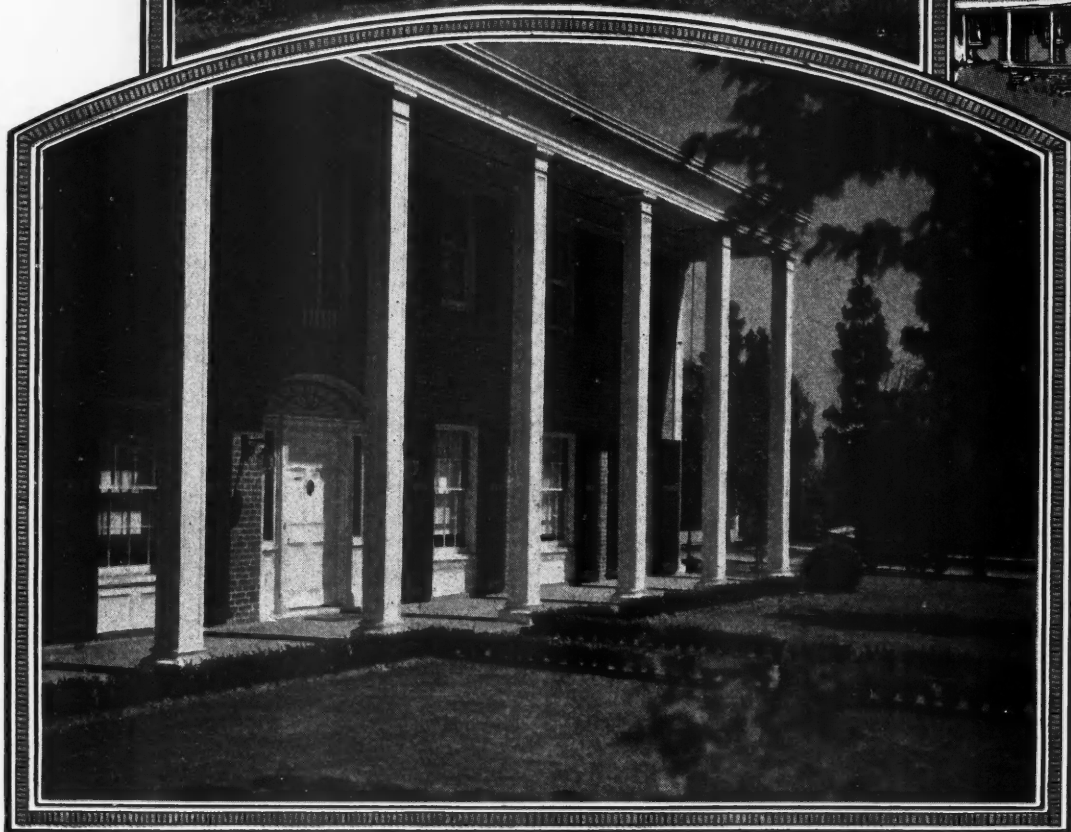
E NTRANCE DETAILS are most important in fixing the architectural status of your new home. The arched opening and massive door, pictured above, typify the old Spanish missions, while the two-story columns and formal balance of shuttered windows fix the lower photograph as of the Southern Colonial or Georgian style.
