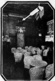
One ILG Electric Ventilator makes this lunch room a joy spot.
