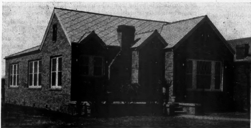
The Fiftieth House Built in Broadmoor by Peyton & Johnson Was Displayed as a "Model" House and Sold Within Two Hours After Being Opened to the Public.
