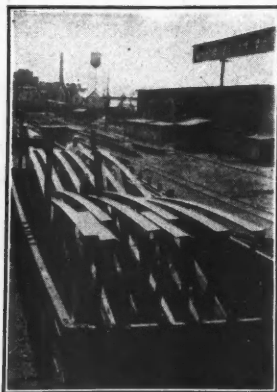
78 foot trusses shipped in two sections for ease in handling and erecting.
