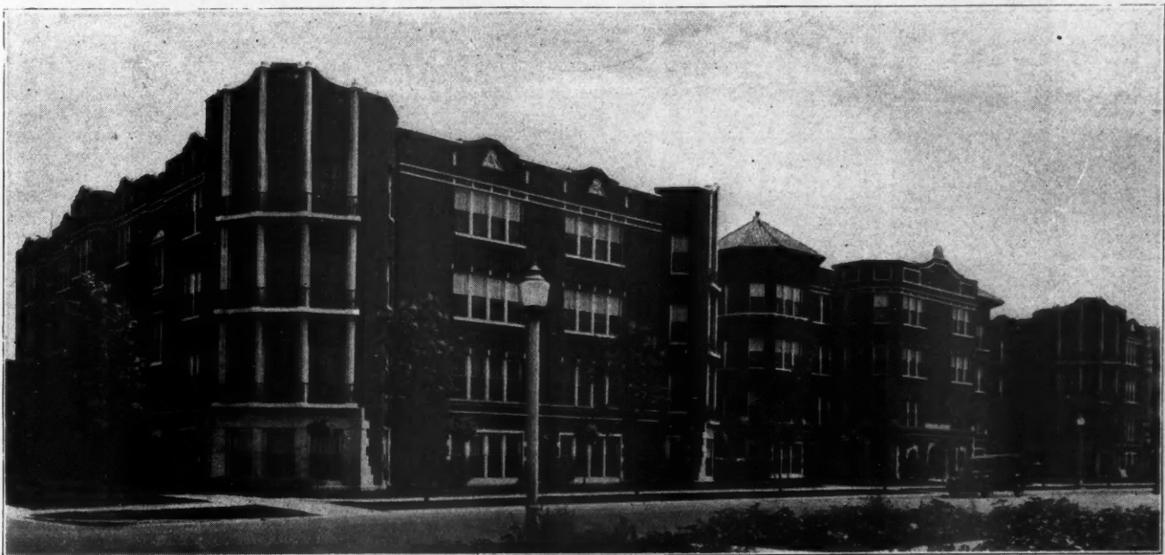
General View of the Ingleside Court Apartments, Located in Chicago's Far South Side. The architecture is exceptionally pleasing and the orientation and daylighting particularly good. The building contains 69 suites of three, four and five rooms and is well finished and equipped. Attention is called to the typical floor plan on the opposite page which shows skillful arrangement. A. C. Lund, Architect.
