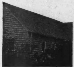
Roof of edge-grain shingles built in 1897. The owner writes: "In all these years I have spent not to exceed $15.00 in repairs and the roof seems as good as ever".
