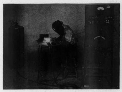
An Operator at Work with the New Atomic Hydrogen Welding Equipment Which Opens Up Entirely New Fields for Electric Welding.
