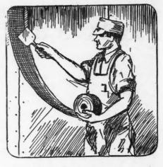
The Joints of Wallboard Are No Longer a Problem with This Sealing and Reinforcing Material Available.
