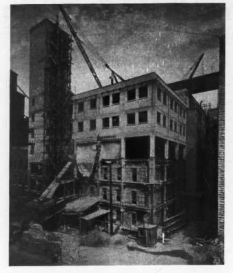
Here Is Shown the Progress of the Construction Work. Two stories of the new building have been completed, the machinery transferred to them and two stories of the old building demolished.
