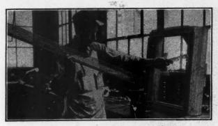
This Simple Little Machine Was Specially Designed to Cut Accurate, Close Fitting Corners on Corner Bead.
