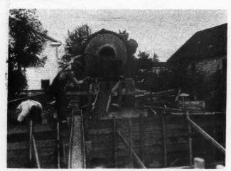
This Combined Truck and Mixer Will Deliver a Perfect Mix Right on the Job Without Delay and at Low Cost.
