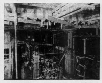
The First Floor of the New Building Which Was Built Entirely Independent of the Rest of the Building and Carried on Separate Columns and Footings,
