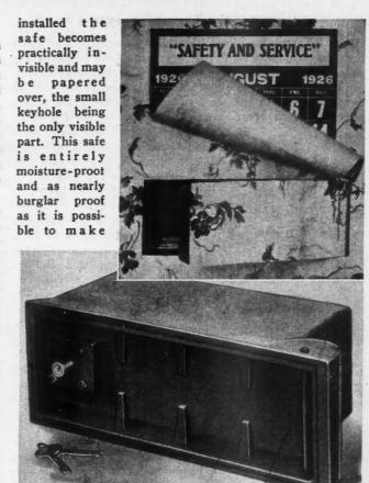
This Safe Can Be Installed in Any Wall and Covered with the Paper or Other Wall Finish so that Nothing but the Keyhole Remains Visible.
