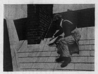
Remove the Old Flashing Around All Chimneys and Dormers and Tack on New Material, Then Proceed as You Would Ordinarily.
