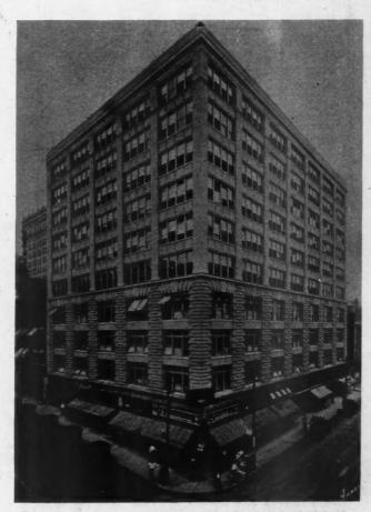
The Use of Light Weight, Burned Shale Aggregate Made Possible the Addition of Six Stories Where Only Four Had Been Planned for.
