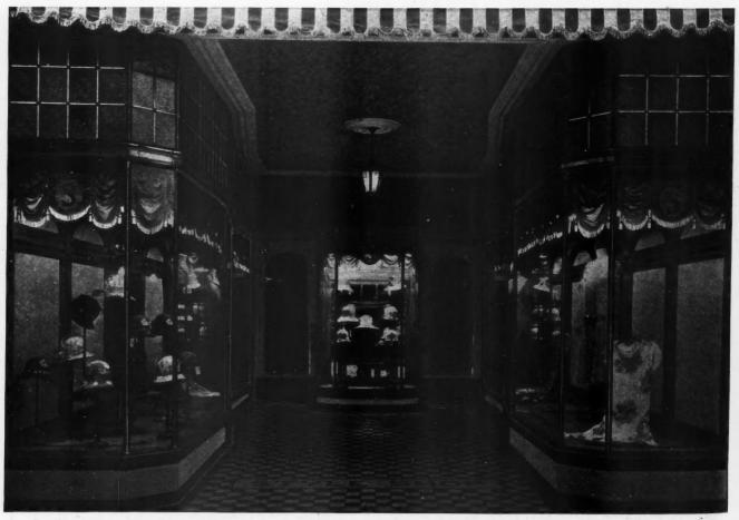
An Attractive Store Front and Entrance Is Here Shown with a Tempting Display of Hats and Gowns. Use is made of a small showcase to separate the two entrance doors and the arcade is widened at this point to allow free entrance and exit. The ceiling above the entrance is a textured stucco with heavy ornamental mouldings. The display windows are brilliantly lit by special flood lights, the bulbs and reflectors being concealed.
