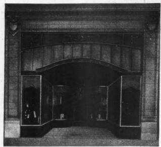
The Features of This Store Front Are Its Free Use of Glass Transom Ornament and the Curved Ceiling Above the Entrance Way Which Extends Out Over the Sidewalk as a Marquis or Canopy. The main display windows face the entrance but at an angle which catches the eye of passersby on the sidewalk.
