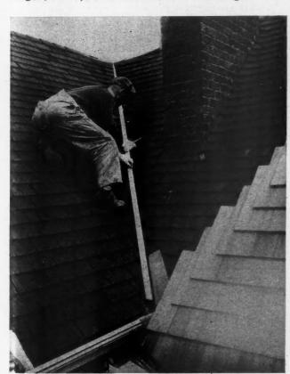
In the Roof Valleys Nail Another Batten in Order to Bring the Flashing on a Level with the Old Shingles and Lay the New Flashing on Top of This.
