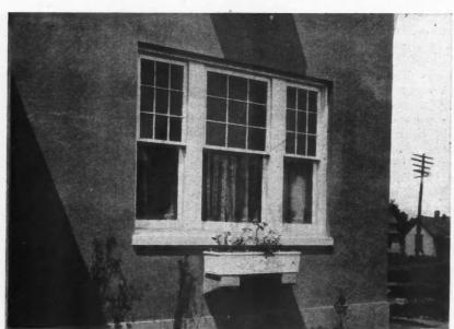
A Severely Simple Wall Treatment. Concrete masonry, on a monolithic foundation, is covered with smooth-textured stucco. The window sill is a precast unit. The window box and its supports are also of concrete.
