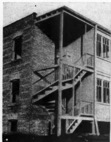
Fig. 1—The Winder Type of Construction with an Unusual Type of Support.
