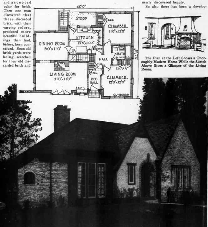
A Pleasing Combination of Face Brick, Slightly Skintled, and Stucco on Hollow Tile with a Wood Shingle Roof, an Effect Peculiarly Adapted to This Particular Design and Showing the Important Relation Between Design and Material.
