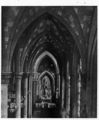
Elsewhere in This Issue Will Be Found an Article on Plastic Paint Decoration. Here is an illustration of its use. A well-known plastic paint material was applied over old plaster and paint in the St. Thomas Aquinas Church, Brooklyn, N. Y., F. Burrell Hofman, architect.
