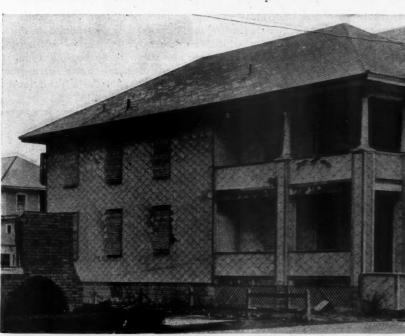
This House, Covered with Asbestos Shingles on Sides and Roof, Acted as a Fire Wall and Protected Two Frame Houses and a Frame Hotel Next to It. The shingles show the effect of the intense heat which burned the window frames, but they ably protected the building.
