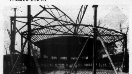
Standard Steel Trusses Which Can Be Immediately Delivered from Stock Are Available for Widths Up to 1021/2 Feet.
