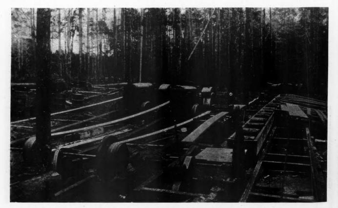
A Portable Sawmill Operated by Two Tractors in East Texas. When one tractor is used the output is from 10,000 to 15,000 feet per day. The extra tractor enables the operator to double his output and may be used, whenever necessary, for miscellaneous hauling, skidding logs and for road work.
