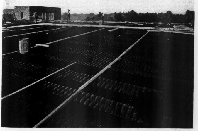
Roof of a Large School Building Under Construction at Ironton, Ohio, Using a Special Ribbed Expanded Metal for the Double Purpose of Form Work and Reinforcement. This concrete roof will be absolutely fire-safe.
