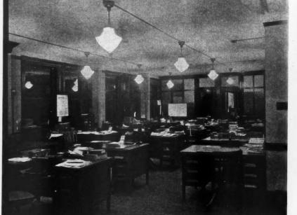
An Office Well Lighted by the Installation of 200-Watt Lamps Giving 2.35 Watts Per Square Foot and an Illumination of 11.6 Foot Candles:
