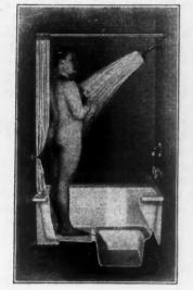
PLATE 10-E Enameled Iron Ware, 44x30 inches to tile in recess, only. Enameled white front. Waste in foot section either right or left hand end. Only one size made.
