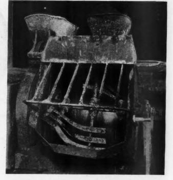
This View Shows the Charging and Discharging Opening of the Mixer Drum of the Mechanical Hoeman on the Pittsfield Building.
