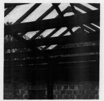
Here May Be Seen the Steel Construction of the Second Floor Ceiling and the Roof. A two-inch sub-roof of concrete was placed on the steel rafters.
