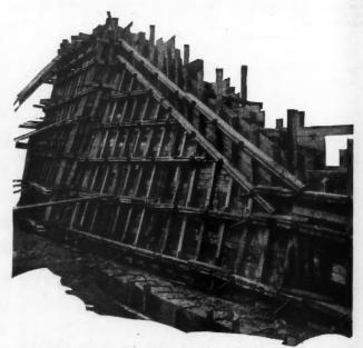
Reinforced Concrete Construction Work of All Kinds Is Greatly Simplified by the Use of Form Clamps Such as Are Being Employed on This Job.
