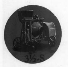
ith 3½-S Tilter — another mixer of 8 seconds charge—furnished with or without power loader. n be had as two-wheel trailer or with 4 steel or hion-tired wheels. Capacity 35 to 50 yds. a day.
