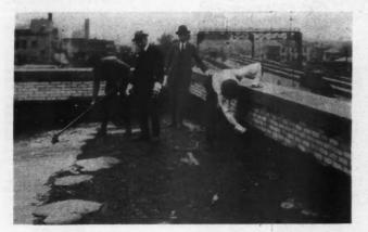
Malleable Asphalt Being Applied on Roof and as Side Wall Flashing on Union Station, Joliet, Ill., Fall of 1925.
