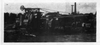
This Paver Is Now Equipped with an Automatic Control Which Relieves the Operator of Over 2,000 Hand Operations Daily.
