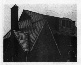
Home on Balfour Road, Detroit, Three Years Old, Showing the Adaptability of Glass Coated Armco Iron Shingles to the Various Angles of Hips, Ridges and Valleys.
