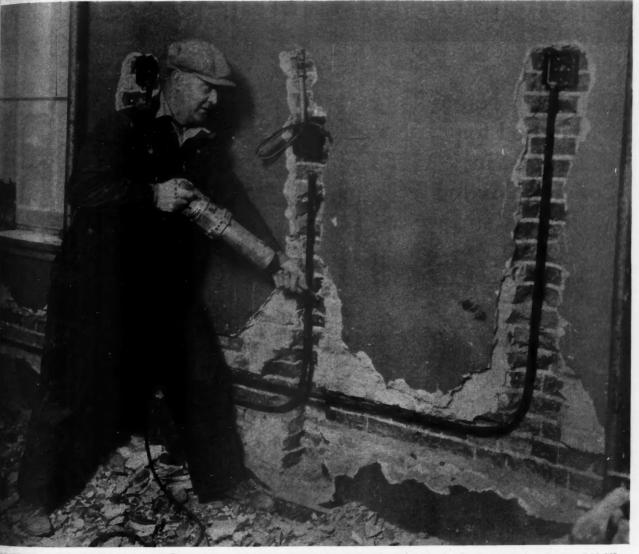
Workman Armed with Electric Hammer Cuts Out Chases for Pipes in About One-Tenth the Time Doing It the Old Way.
