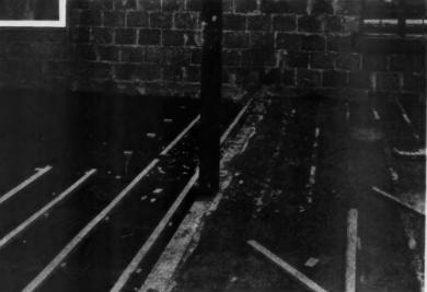
This Shows How the Concrete Floors Were Laid Over the Metal Lath with Sleepers Imbedded for Nailing Down the Hardwood Floors.
