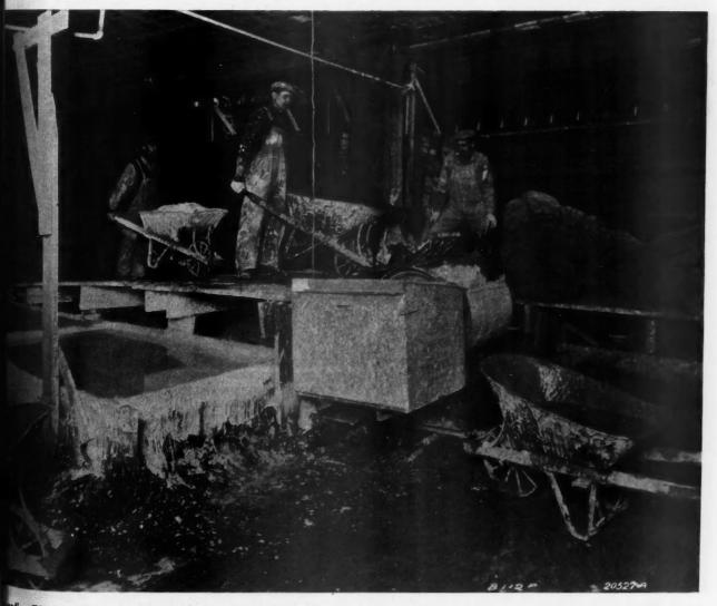
Platform Built to a Level with the Top of the Mixer Greatly Facilitated Loading on the Pittsfield Building Job.
