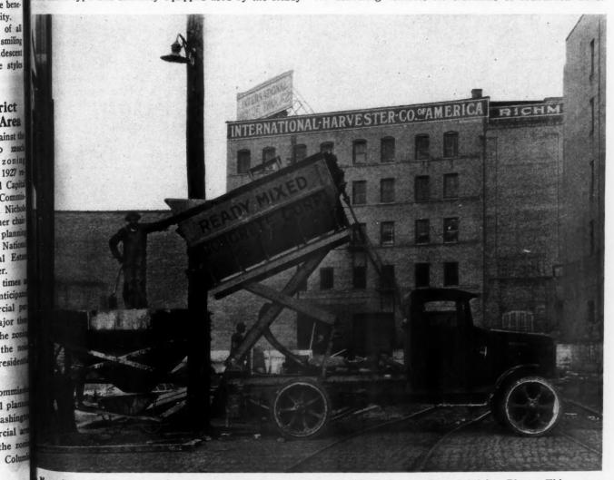
Kiny Cities Builders Are Now Buying Their Concrete Already Mixed, from a Central Mixing Plant. This motor truck mounted equipment delivers the mixed concrete to the job.
