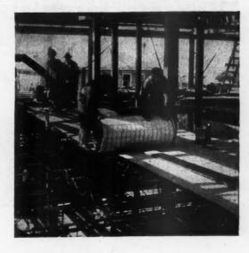
STEELTEX for Floors is an extra-heavy, specially-processed backing locked to an electrically-welded steel fabric similar to National Reinforcing. The latter has been used for many years for all concrete, terrazzo, or gypsum floor work wherever wood forms are desirable. Send the coupon for complete details.
