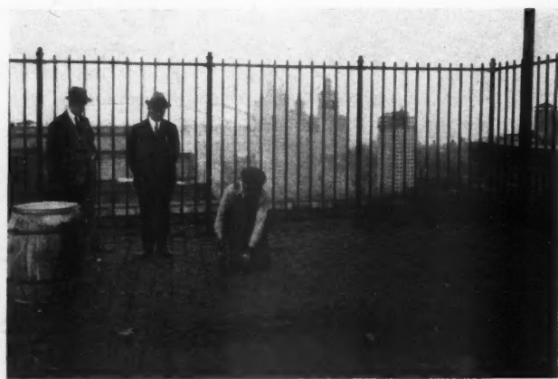
In Making a Permanent Repair of This Tile Roof the Workmen First Broke Out All the Original Setting Material That Had Become Hard and Brittle.
