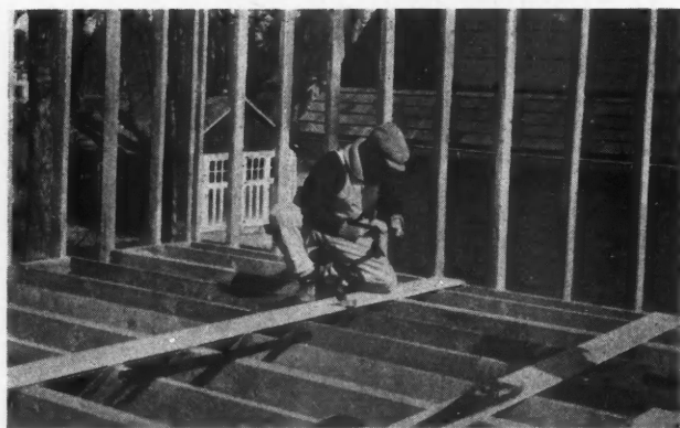
The Bridging Strips Come in Straight Pieces Which Are Bent on the Job and Are Adjustable to Variations in Size and Spacing of Joists.
