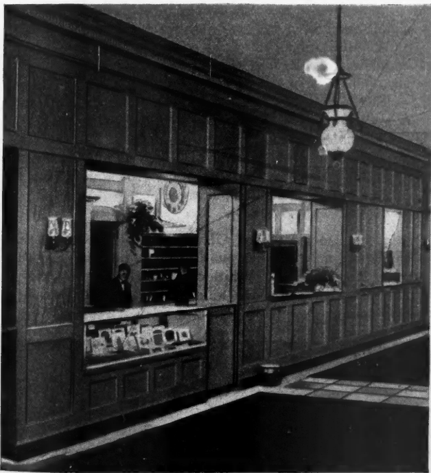
Entrance lobby with Pine panelled walls. Millwork supplied by M. T. Blasingham & Co. and C. M. Baylor and Co.; Shevlin Pine by McEwen Lumber Company; all of Norfolk, Virginia.
