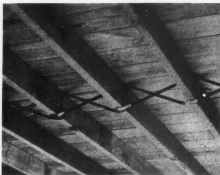
This Type of Steel Bridging Makes an Integral Connection Between Three Joists.
