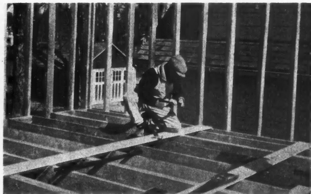
The Bridging Strips Come in Straight Pieces Which Are Bent on the Job and Are Adjustable to Variations in Size and Spacing of Joists.
