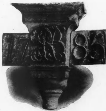
This Copper Leader Head Dates Back to 1785 and Has Given Perfect Service for Many Generations.
