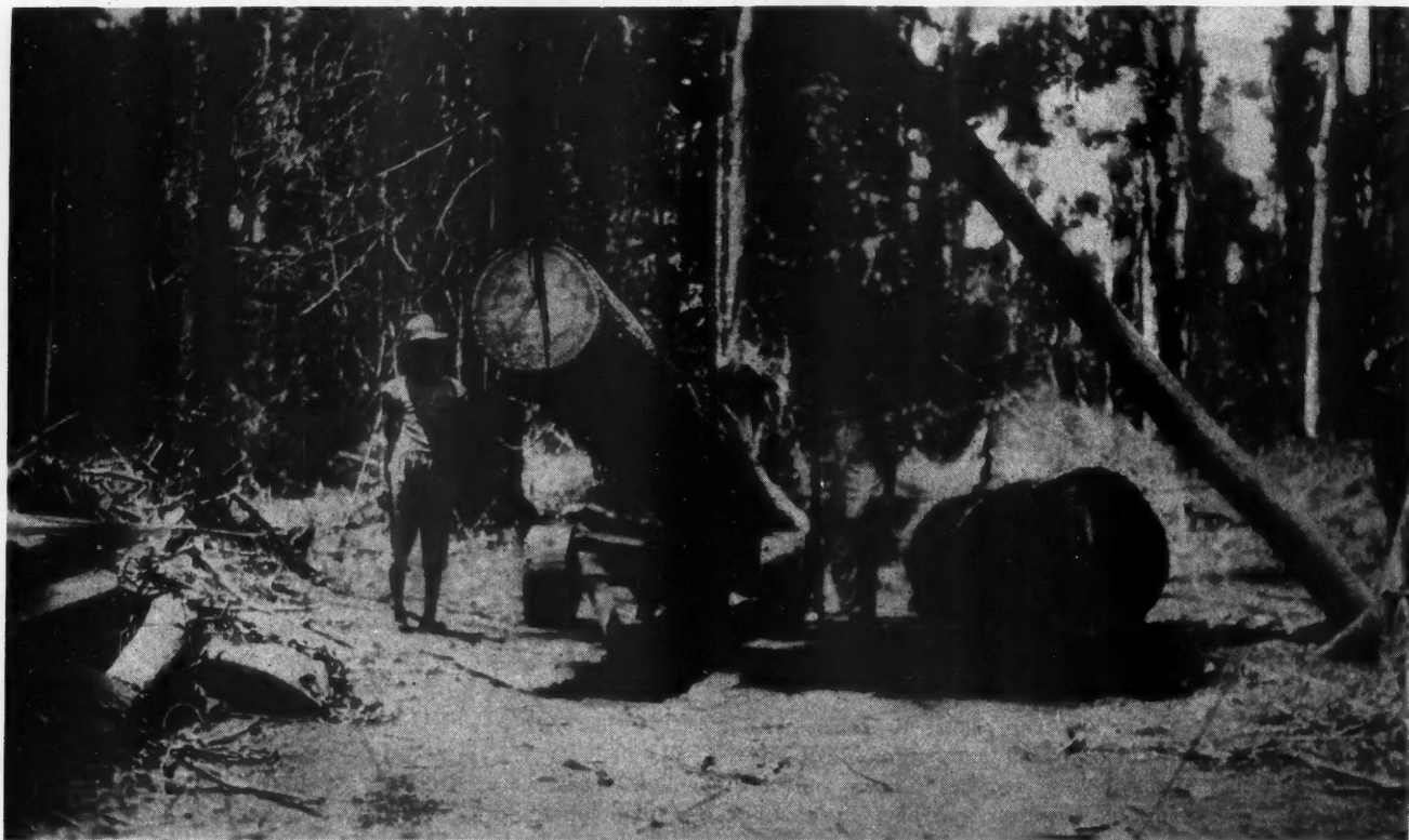
Loading the Large Philippine Hardwood Logs in the Forests of the Philippine Islands. These logs are hauled first to a railroad and then to the mills or rivers.
