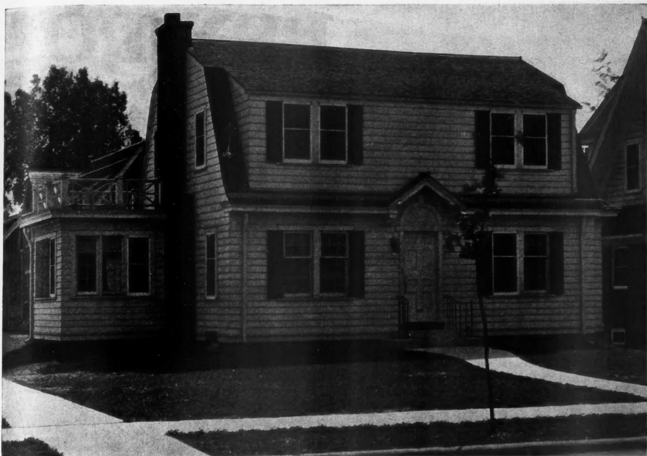
A Typical Hercules Built Home, Constructed from Plans Which Are Furnished to All of the Subscribing Companies. Special designs are also prepared for prospective builders and these become available to all subscribers with the limitation of building but one house from these plans in each city.
