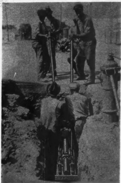
A Pipe Pushing Jack Which Grips the Whole Surface of the Pipe and Avoids Crushing and Distortion.
