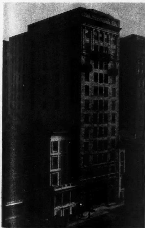
The Old Building to Which It Was Desired to Add Six Stories Was Not Designed to Support This Additional Weight.
