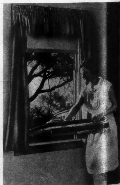
Any Double-Hung Wood Sash Can Be Equipped with This Hardware so That It Will Tilt in for Cleaning.
