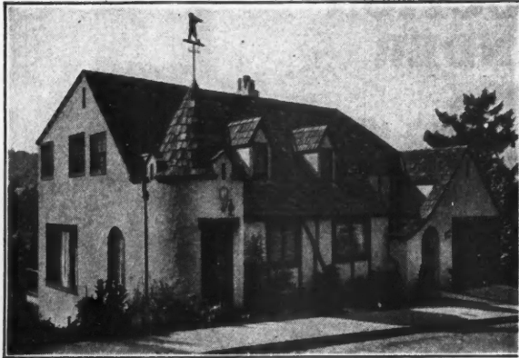
House on Portland Heights, Portland, Oregon. Cash and Wolf, Architects, Harry Phillips, Contractor. Roof of Cabot's Creosote Stained "Shakes." Exterior Woodwork finished with Cabot's Creosote Stains, Insulated throughout with Cabot's Quilt.
