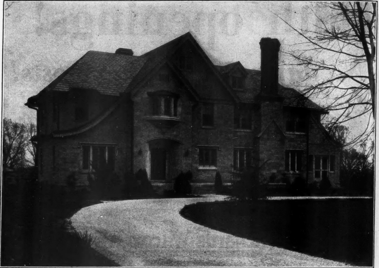
Residence, Memphis, Tennessee. Sieg & McDaniel, Architects Built of Variegated Indiana Limestone Random Ashlar
