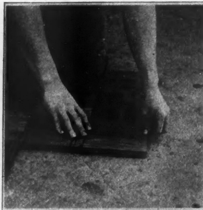
The Final Steps in the Process of Laying Wood Block Flooring. This is so simple and rapid that labor cost is materially reduced, bringing parquetry flooring within the range of any flooring estimate.
