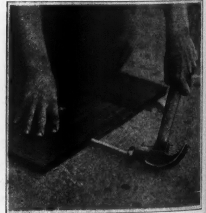
The Final Steps in the Process of Laying Wood Block Flooring. This is so simple and rapid that labor cost is materially reduced, bringing parquetry flooring within the range of any flooring estimate.
