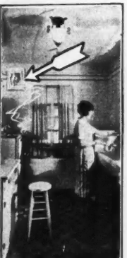
Another typical installation of the built-in ILGAIR Electric Ventilator featured in a model home.
