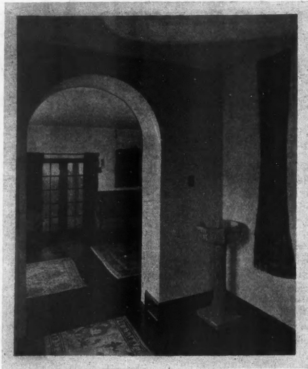
In Modernizing Wonderful Results Can Be Obtained by the Use of Metal Lath and Plaster to Introduce Arches, Niches and Vaulted Ceilings.
