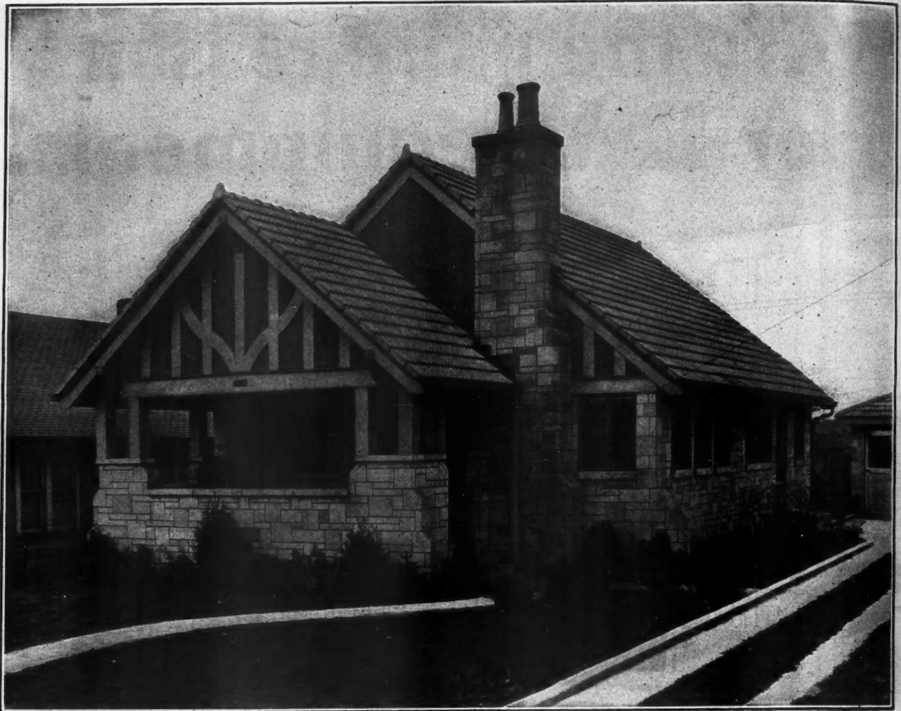
Residence, Bedford, Indiana. Old Gothic Random Ashlar is entirely practicable for construction of this type, although naturally its appeal is greatest in houses of a somewhat larger type.
