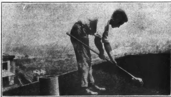
This Material Can Be Applied with a Brush by Any Workman to Any Type of Roof.
