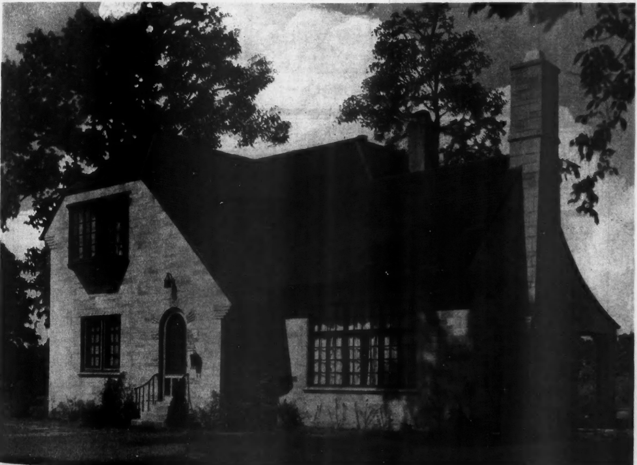
A Four Inch Veneer of Indiana Limestone Gives This Residence an Impressive Appearance. A. Frank Ranahan, Jr., owner, Edgewood Grove, Ind.; Johnson, Miller, Miller & Yeager, architects, Terre Haute, Ind.
