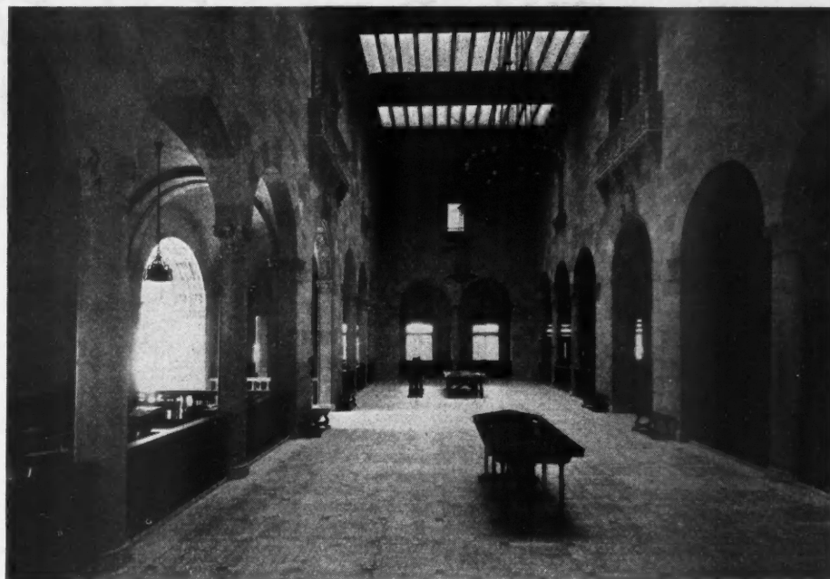
A Public Lobby, with Richly Carved Balconies at the Sides and Ends and Walls of Toned Travertine Stone, Extends Across the Building.
