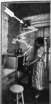
Model Home in a large Chicago department store where the ILGAIR Ventilator was one of the outstanding kitchen features.
