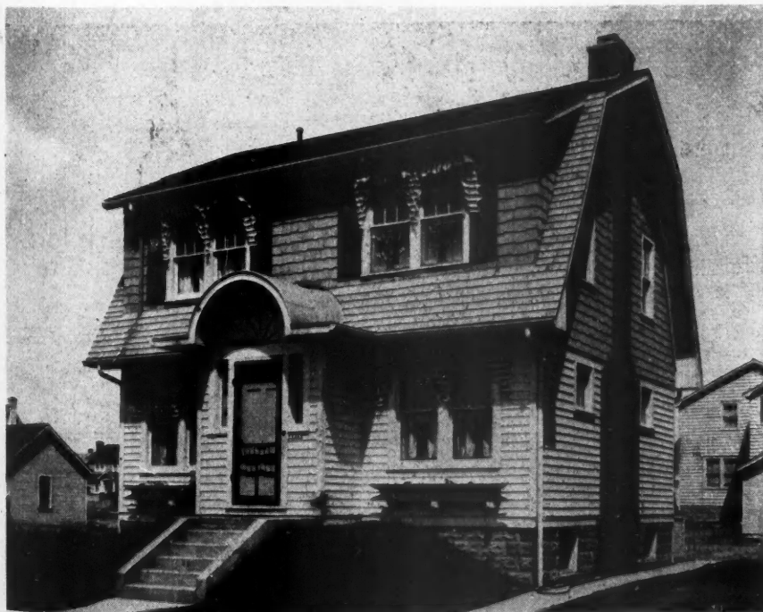
A Few Small Roof Changes to Create a Dutch Colonial Design and a Few Changes in the Windows Made All the Difference Between This House and the One at the Top of the Page.
