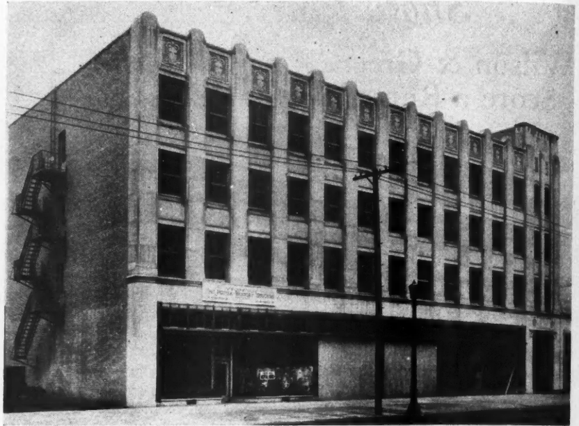
The Upper Carnegie Building, Cleveland, Ohio, Is the First Commercial Store and Office Building of Arc Welded Steel Construction.
