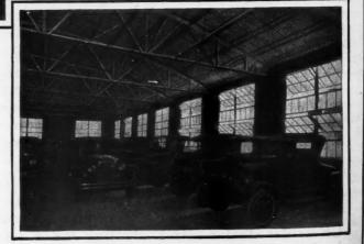
(In Oval) E.S.Koon Warehouse, Asheville, N.C. Massillon RoofTrusses in position ready to receive purlins. S. Sternberg & Co., Engineers.
