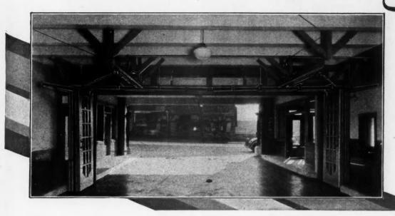
This entire installation—doors, hardware and power—is R-W equipment. The four entrance doors or the four exit doors operate independently—or all eight doors may be opened and shut simultaneously—from any part of the garage or office, by simply pulling a cord or pushing a button, several of which are conveniently located.
