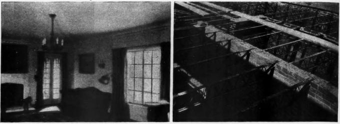
Doublemesh Herringbone Metal Lath-the ideal base for firesafe, permanent, crackless plaster.
