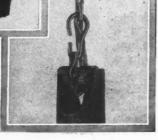
A coil spring is slipped over the end link of the chain before it is fed into the window casing. After hooking weight as shown above, the coil is inserted into the bore of the sash. For two hole sash the coil is inserted into the upper bore.
