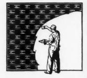
The plasterer doubles right back over the scratch coat, saving the time and labor ordinarily required to remove and re-erect scaffolding.
