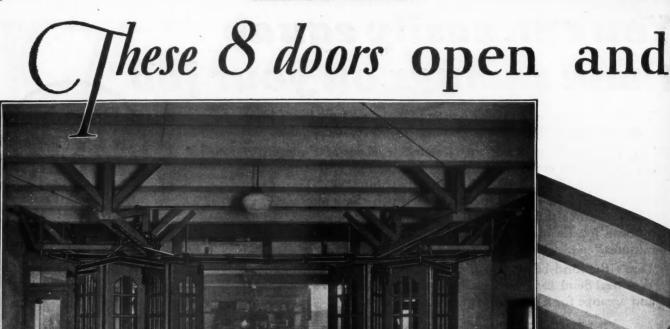
Capitol Garage, Kansas City's largest, NEVER keeps a patron waiting. Only R-W equipment assures such service. These doors close weather tight. They open INSIDE so ice and snow NEVER hinder operation. A simple adjustment allows for swelling or shrinking of doors. No center posts. The same R-W advantages for doorways up to 30 feet wide.
