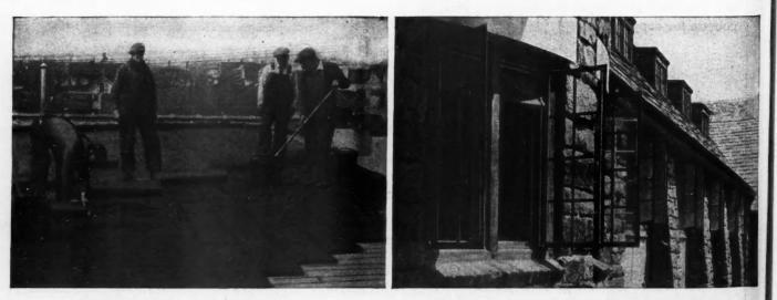
**Rigideck**, the light weight, fireproof roof deck. Laid like boards. Made of rust-resisting Armco Ingot Iron.
