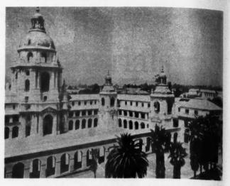
City Hall, in Pasadena, California, Roofed with Lead Coated Copper Which Will Last Indefinitely.
