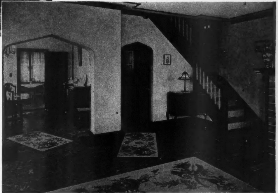
Armstrong's Linoleum throughout this Model Home; red tile in entrance hall; Italian Handmade Marble Inlaid, with black border, in living-room and dining-room; Embossed Inlaid design in breakfast room, kitchen, and back porch; taupe Jaspé in bedrooms.
