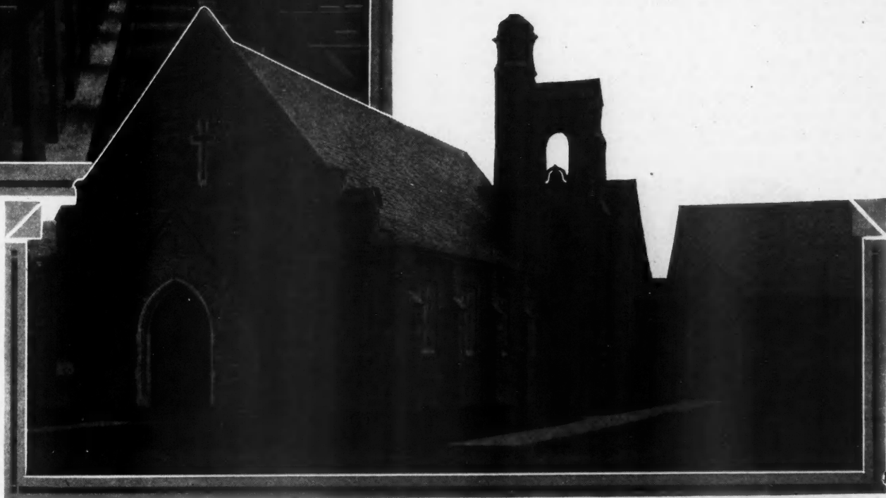
Exterior and Auditorium Views of the Methodist Episcopal Church, Trainer, Pa. Thoralf M. Sundt and Bruce C. Wenner, of Philadelphia, Pa., architects; William Provost, Jr., Chester, Pa., general contractor. This church, which cost $75,000, was awarded first prize of $1,000 in a nation-wide competition for average sized church buildings.
