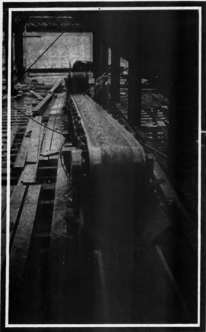
24-Inch Belt Conveyors, 60 Feet Long, Handling Wet Concrete.
