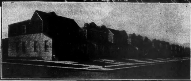
2700 Radia Electric Heaters were specified for bathrooms in above development, Flatbush Centre, L. I.
