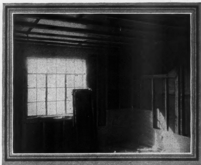
Sidewalls and Ceilings Are Thoroughly Insulated.
