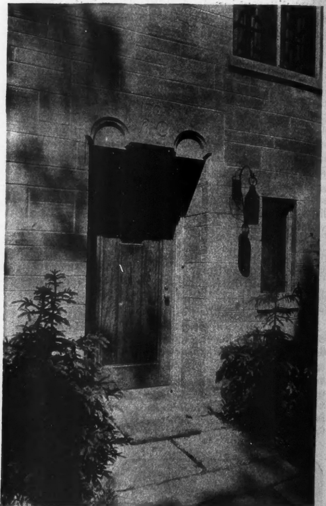
Here is the entrance to a home built of beautiful Indiana Limestone Random Ashlar.
