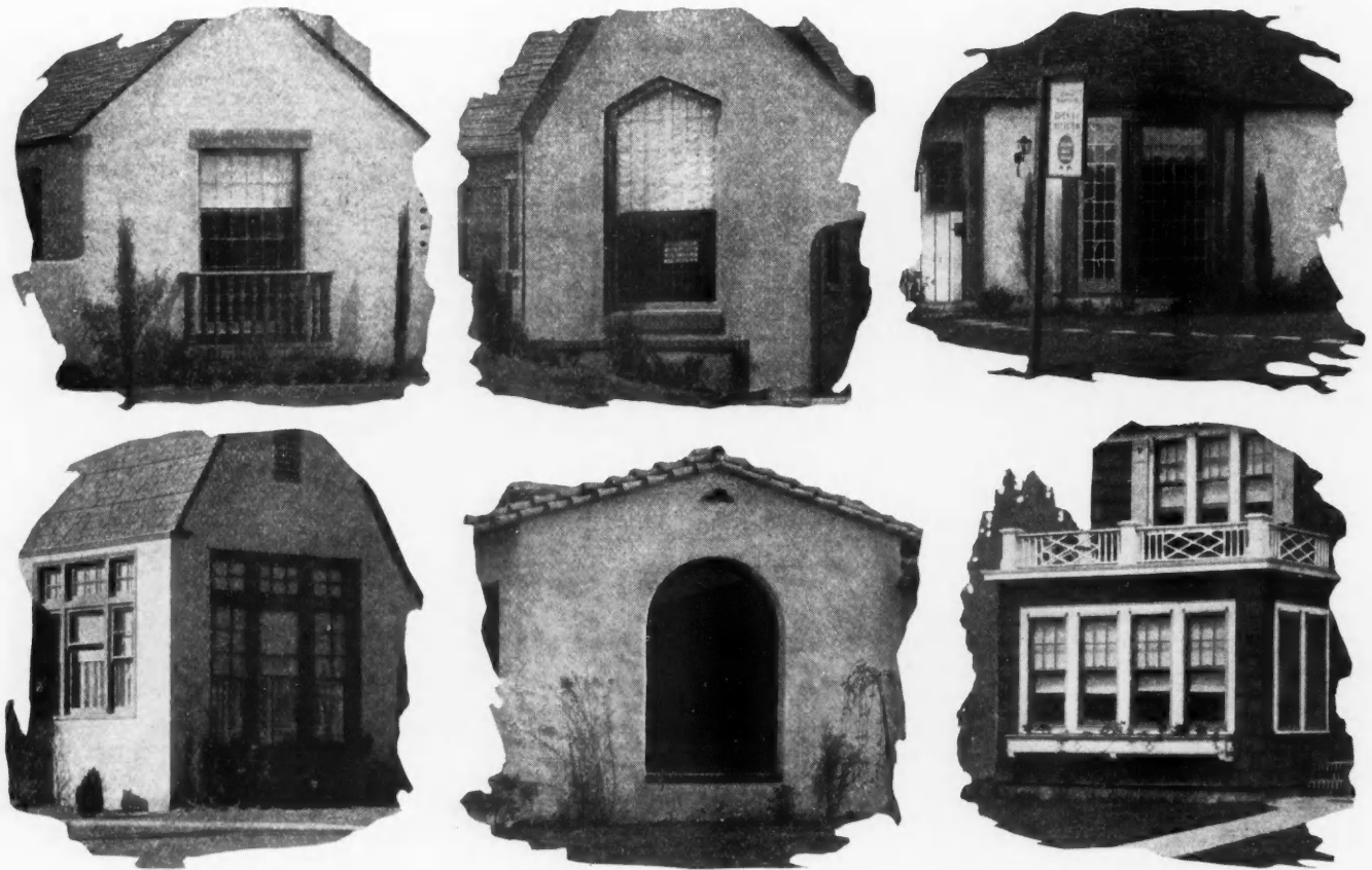
H ALF a Dozen Window Design Ideas Gleaned from East and West. Studio-Windows, Picture-Windows, Bay-Windows, and Mullion Groups are Popular Today.
