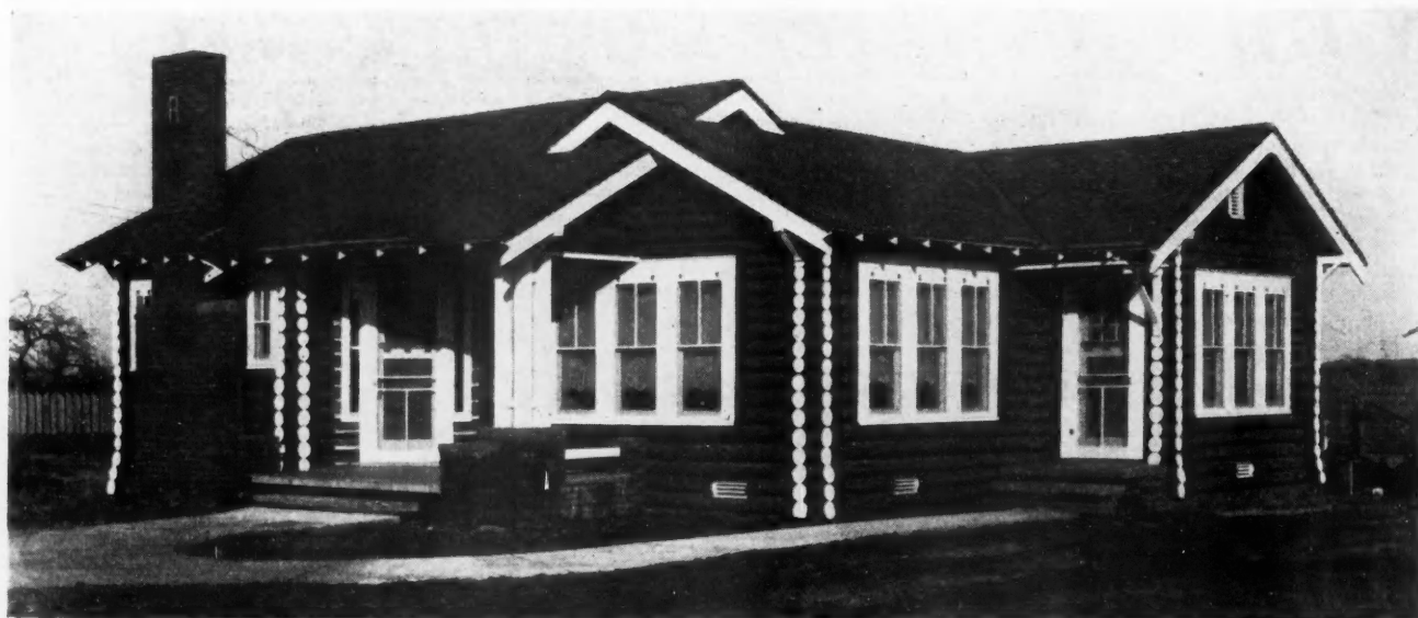
Although Built of Pine Logs in Regular Log Cabin Style, the Interior of This Home, Built by E. D. Maxwell, Marlin, Texas, is Finished Exactly Like the Conventional Dwelling.
