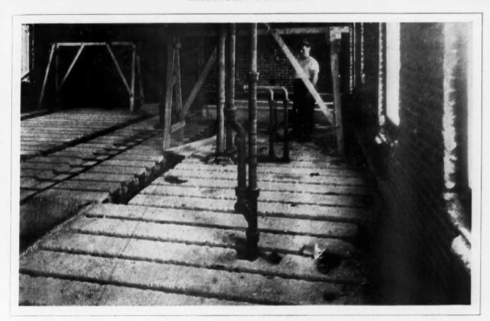
Fig. 5. Miller Units Assembled Before Concrete Topping Is Placed. When open space between ends of units is filled with concrete, projecting bars are embedded and anchored.
