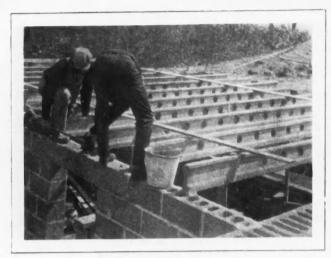
Fig. 6. Bedding Joists in Mortar. These joists may be cut to length and handled almost as easily as lumber.
