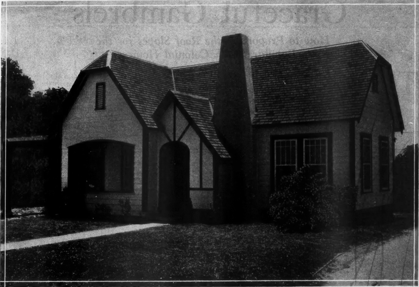
GUARANTY BUILDING CORP., Architects & Builders, San Antonio, Tex.
