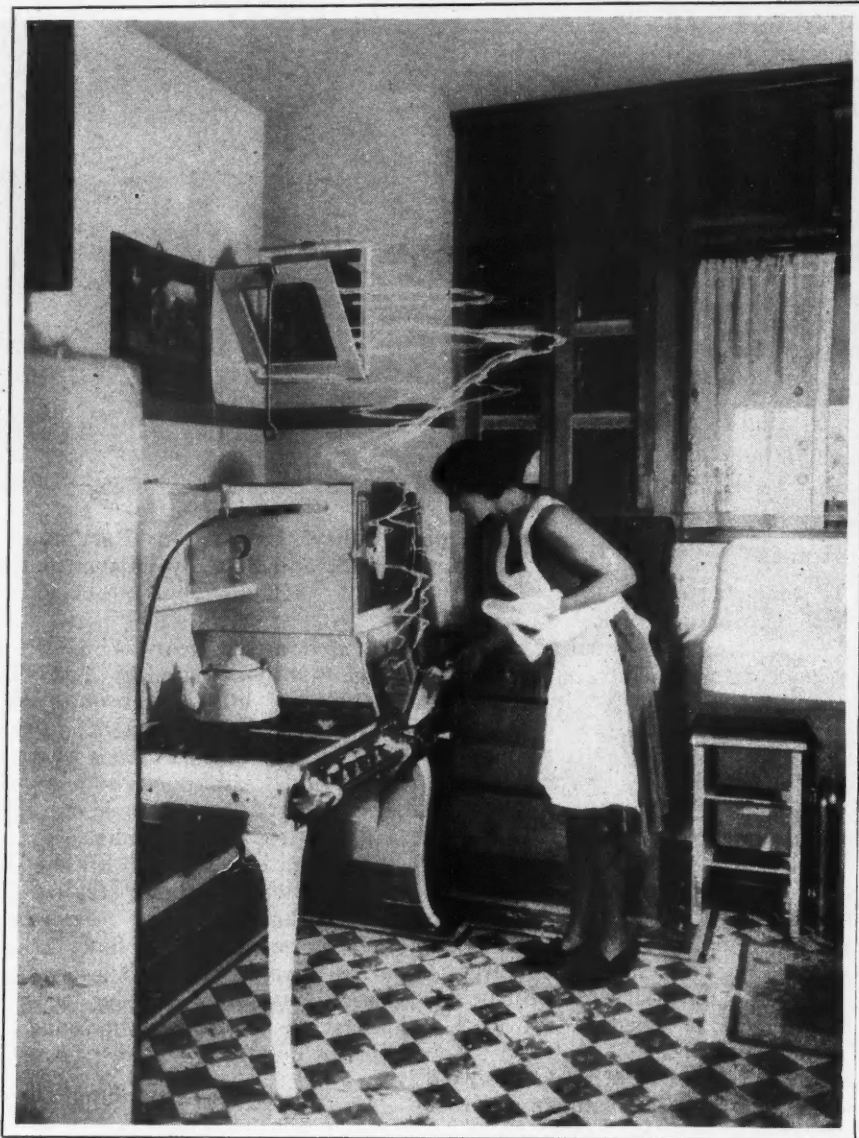
Electric Fan Installed in Outside Wall.
