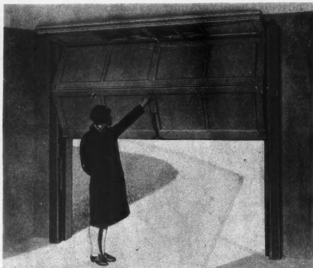
A New Garage Door Which Folds Up Inside the Opening Is Easily Operated by Anyone.
