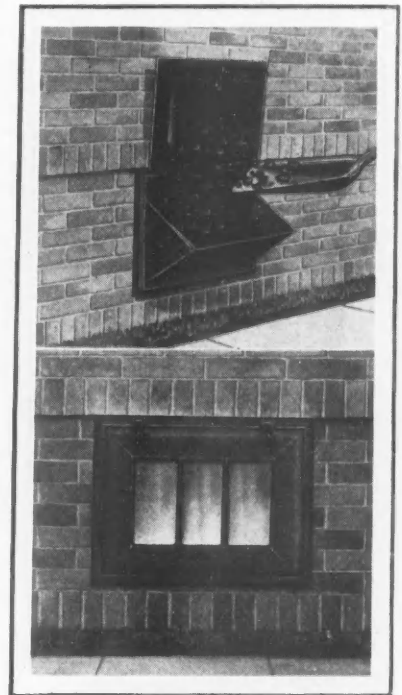
The Plate Glass in These Coal Chutes Has Proven Stronger Than Wire Glass.
