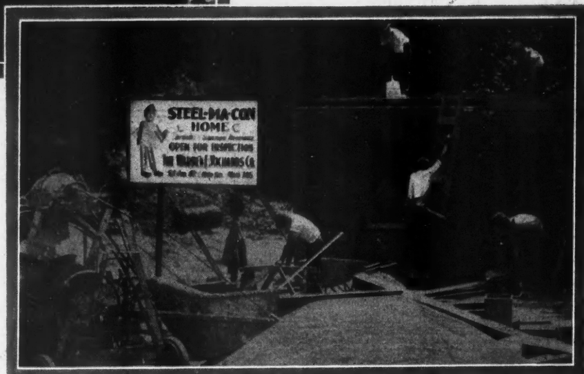
To Right: Workmen Lay- ing the Concrete Second Floor of the Cincinnati Enquirer Model Home.
