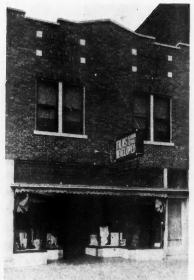
There Is an Opportunity for the Contractor in Modernizing Store Fronts.
