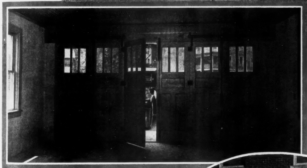
Doors That Slide and Fold Are Installed to Work Either Inward or Outward, and Are Equally Successful for Small Private and Large Public Garages.
