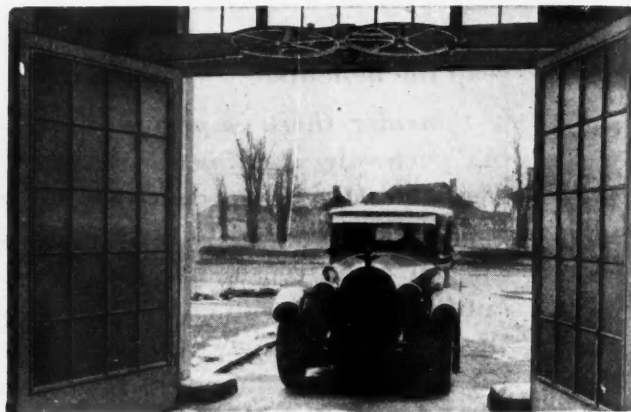
Automatic Garage Door Openers Afford Control from Any Number of Remote Points.
