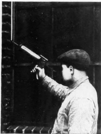
It is a Simple Matter for Any Workman to Apply This Calking Cement with a Gun.
