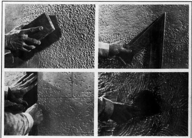
The Finer Texture Effects Now in Vogue Can Be Secured in This New Color Plaster with Surprising Ease. Pictures at upper left and upper right show a brush stipple and its partial smoothing down. A draftsman's triangle makes an excellent tool for this purpose. A picture at lower left illustrates the splendid Travertine effect gained with this new product and a whisk broom wave at the right. Above, a finished room.
