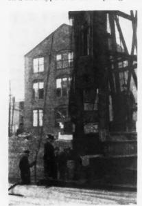
The New, Hollow Concrete Piling Driven by a Steam Hammer, Showed No Spawling or Booming.
