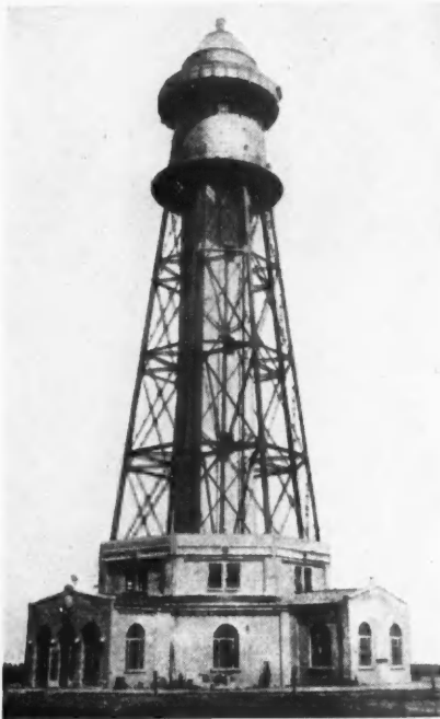
The World's Largest Mooring Mast with a Substructure of Concrete Block.
