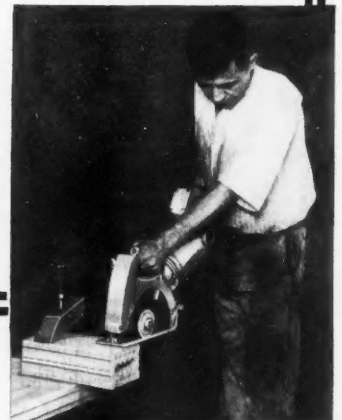
Cutting tile—good, clean cuts, no breakage
