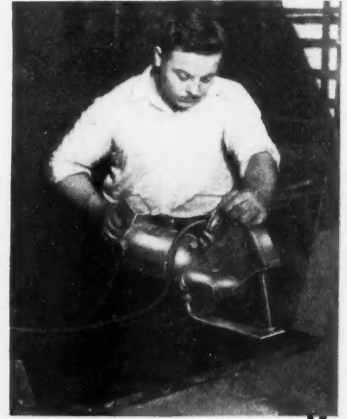
Cutting marble facing one inch thick
