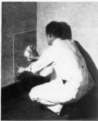
Applied Like Wallpaper with a Special Adhesive.
