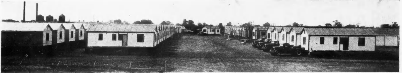
House Factory Assembly Yard at Long Island City.
