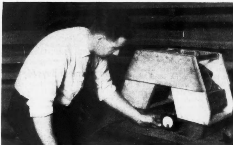
Testing a Weld by Means of the New Magnet and Meter Method Which Does Not Destroy the Weld.
