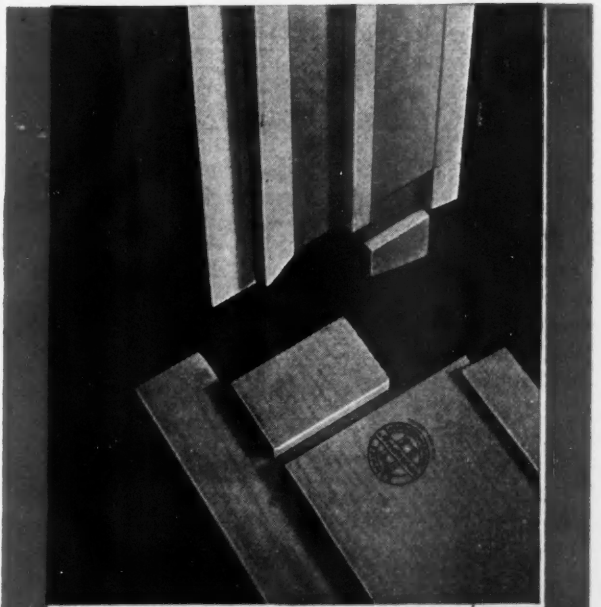
Photograph showing sill and jamb dados before joint is closed.
