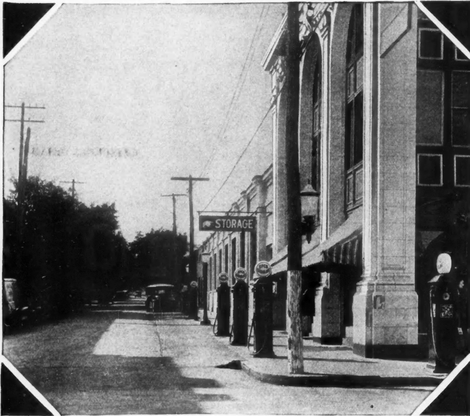
High - Early - Strength concrete approaches to garage and gasoline tanks of Epley Garage Co., Gettysburg, Pa. Universal Atlas methods and cement used. Peters Cement Products Co., Gettysburg, contractor.
