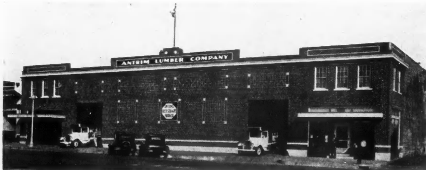
The New Enid, Okla., Plant of the Antrim Lumber Company in Which Attractive Appearance Is of Equal Importance with Efficient Layout.
