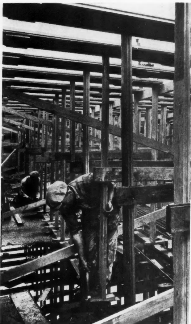
Step 1—The 2 by 6's are used for Shoring and Forms.
