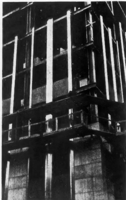
Workmen Placing Limestone and Metal Facing on the Empire State Building.
