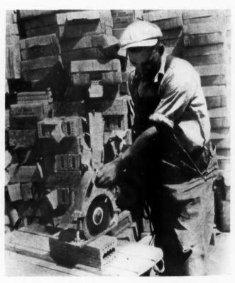
Cutting tile, brick, or stone with an electric saw is the only practical way. In addition to being many times as fast, the electric saw saves material and insures an accurate fit.
