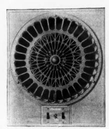
An Electric Element and Fan Inconspicuously Built into the Wall for Heating the Room.
