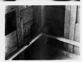
PARTITIONS and stairs built before walls (at left) by Enterprise Bldg. Co. Above, John Haeber's Milwaukee method of fixing grounds at corner.
