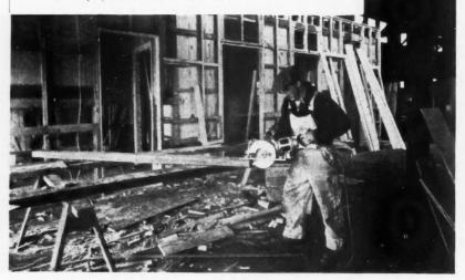
Electric hand saws are from 7 to 10 times as fast as "muscle" hand saws. They will rip a 2-inch pine plank 6 feet long in 30 seconds.
