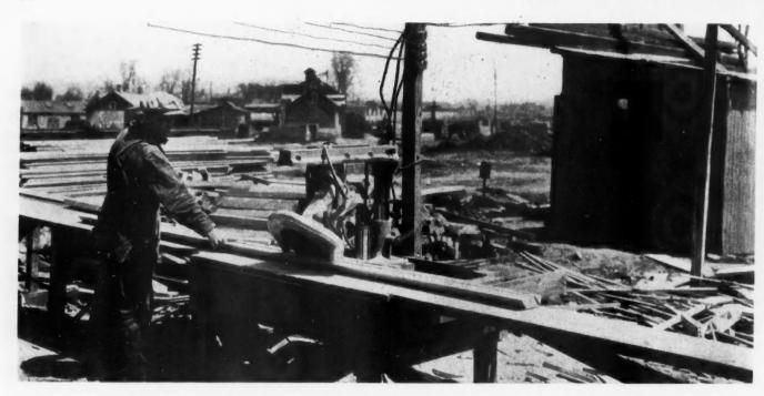
On concrete form work the power saw has reduced carpentry cost 50%. It is used to rip, cross-cut or bevel all columns, end beams, battens, stair-risers, wedges, shoring, spreaders, etc., and speeds up the entire job.
