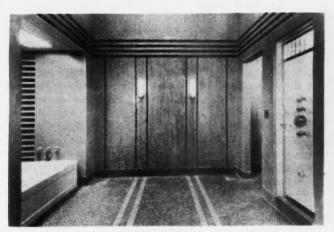
New Individual Colors and Textures Have Been Developed in Rubber Floor and Wall Coverings.
