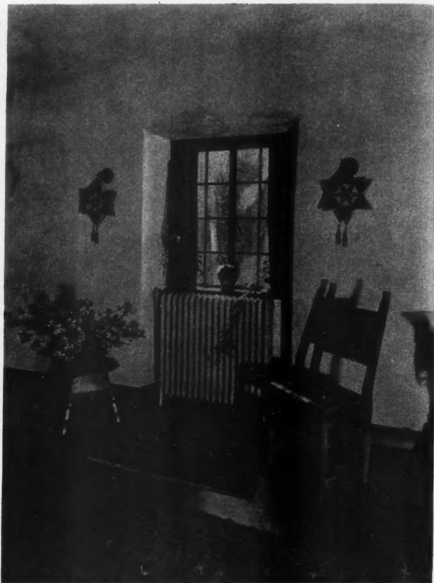
Recessed Radiator Below a Window Indicates Careful Planning.
