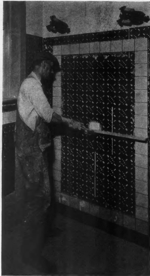
With a Straight-edge and Hammer It Is a Simple Matter to True up Tile Which Is Set by This New Method.
