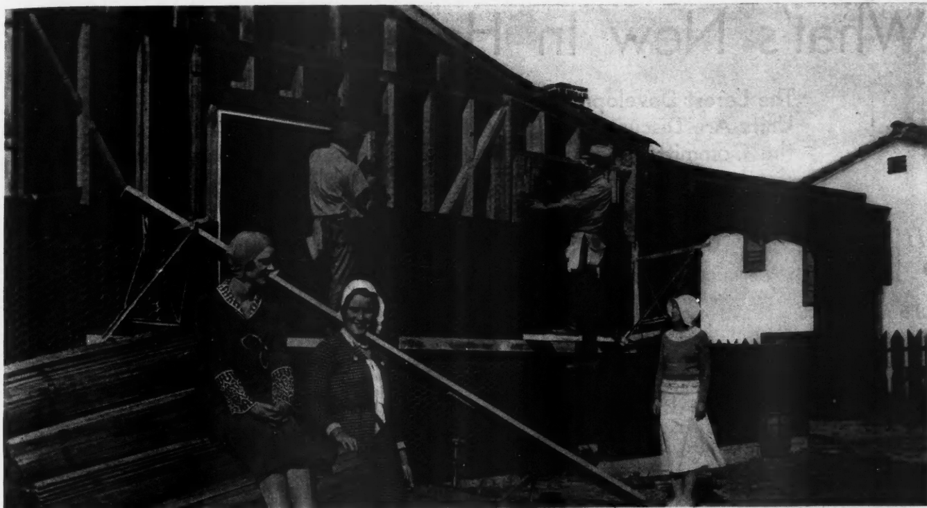
Applying Backing for Stucco Exterior. The posed action photograph interests the public in home-building methods
