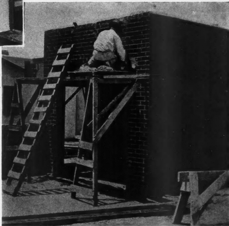
Gypsum Plaster Base in Position with Metal Lath Corner Reinforcing, Dining-room Alcove. Builder, W. E. Rudasill; plaster contractor, R. L. Henderson.
