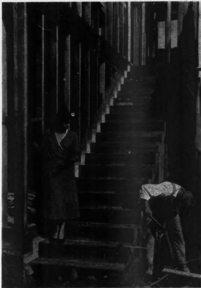
An Especially Good View Which Brings Out Important Features of Stair Construction and Immediately Catches the Interest of the Public. The framing methods, cross bracing, sill construction and other details may be explained and prospective buyers told why they can expect a satisfactory and lasting job
