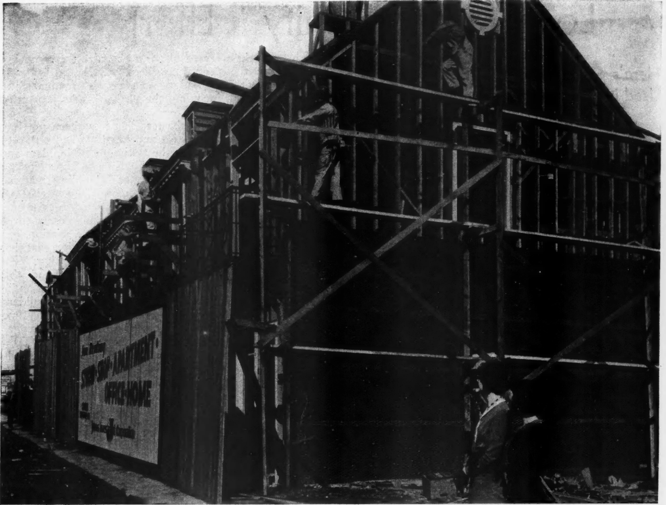
Framing Details for Studio-Shop-Apartment Structure Being Erected by Janss Investment Corp. of Los Angeles
