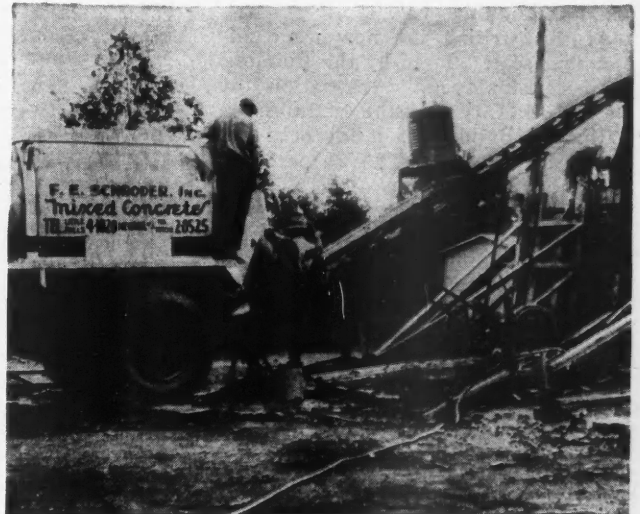
Truck Mixer Discharging Concrete On Belt Conveyor.
