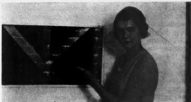
How Inside of Stucco Wall Looks: Note wire reinforcing under paper backing. Braced frame is emphasized
