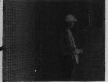
Sheets of Ribbed STEELTEX Lath for interior plaster are nailed direct to the wood frame studding. Rib stiffeners, fibrous backing and wire reinforcing mesh give Ribbed STEELTEX board-like rigidity.
