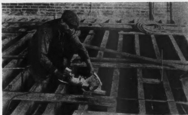
Notching joists for conduits with an electric hand saw.
