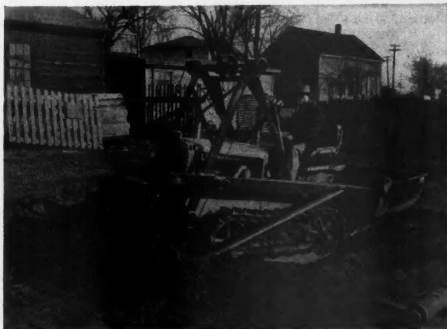
Above—electric drills and hammers are constantly useful. At left—how one contractor cuts curbs with a tractor.
