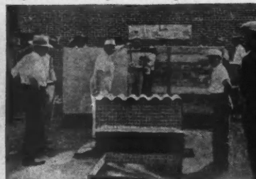
(Below) STEELTEX and one inch cement applied direct to studs is twice as strong as diagonal sheathing and siding.
