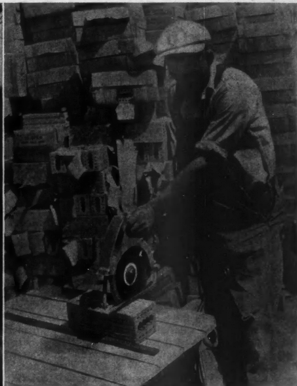
At left—advance in excavating and earth hauling equipment has been great. At right—using a hand power saw to cut tile quickly and accurately.
