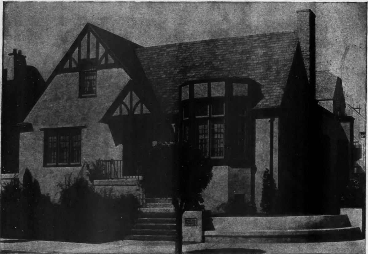
Park Way Terrace, San Francisco, glazed with Libbey-Owens-Ford Quality Glass. Architects—Kent & Hass
