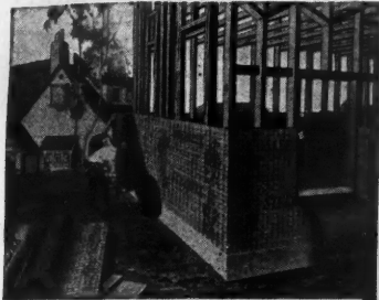
STEELTEX 38-16 is wrapped around in shingle fashion, and nailed direct to wood studding. STEELTEX has three-ply water-proofed membrane backing integral with wire reinforcing mesh.
