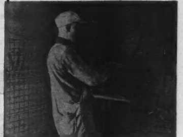
Ribbed STEELTEX Lath holds the wet plaster with instant bonding action. Plaster flows under and around the galvanized, copper-bearing wire reinforcing mesh which becomes completely embedded,—giving lifetime walls and ceilings.
