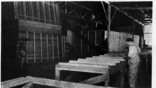
Assembling the roof frames in table top forms
