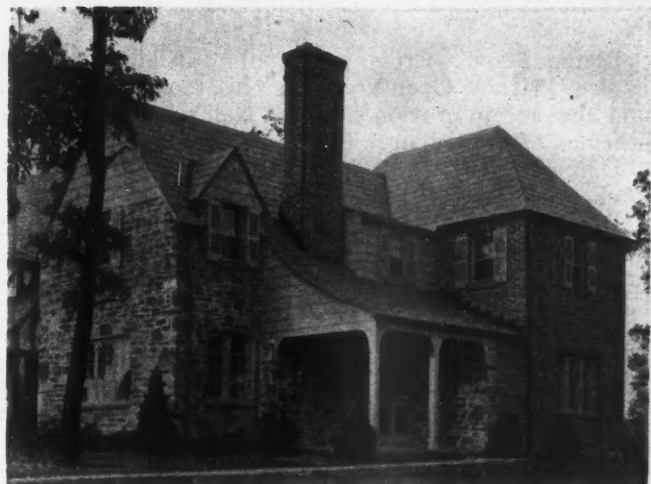
Another C-1 type house with exterior finished in stone, brick, and wide siding. Open porch was specified.
