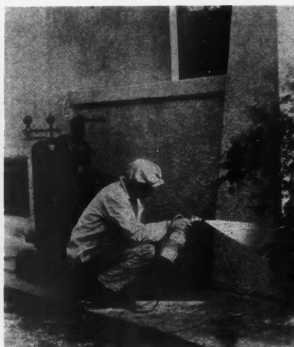
Spray paint equipment has a wide use in refinishing stucco exteriors.
