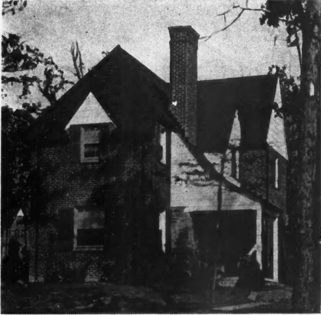
Type C-11 is somewhat smaller than the basic plan, being only 22 feet wide, but follows its general arrangement.
