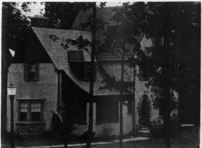
Although following the general basic plan, this house, type C-2 has a third story, and is modified with an enclosed porch. Third floor layout is shown on page 34.
