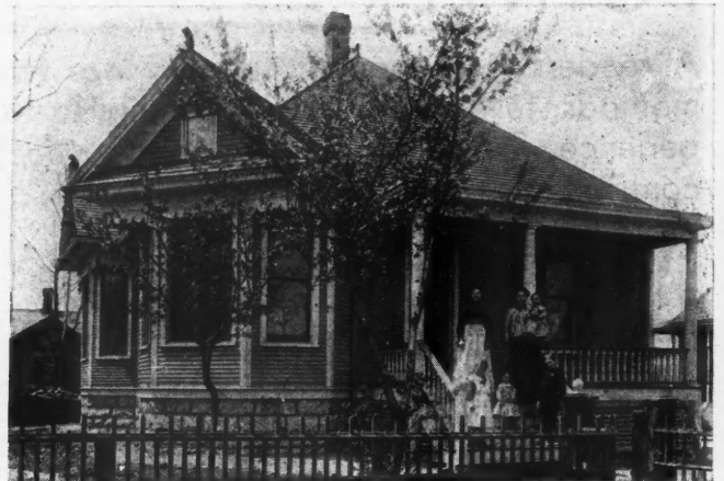
BEFORE MODERNIZING —An old picture showing the old fashioned house before it was covered with new brick veneering.
