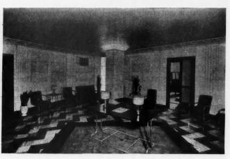
An interior finished with new material which is non-inflammable, sound absorbent, permanent and available in many colors and textures.
