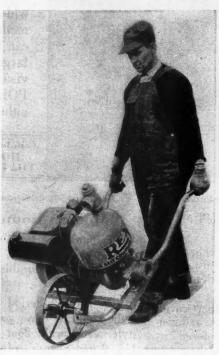
New portable pump will handle 20,000 gallons per hour. Weighs only 385 pounds.
