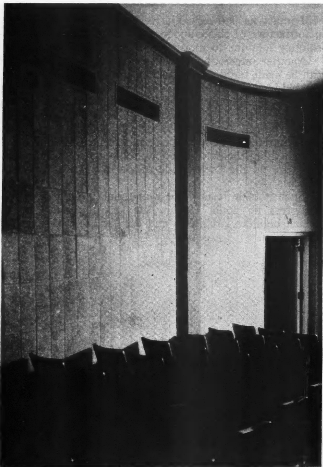
AUDITORIUM of the General Motors Building showing use of 8x8x16-inch light weight concrete masonry units laid on end to form interior walls. Vertical and horizontal mortar joints are continuous. A finish of buff portland cement paint was given.
