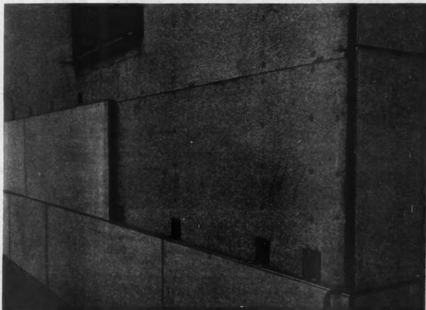
One-inch panels of Colotex insulation used under Macottaglasiron panels for exterior insulation and surfacing of the Stran-Steel Good Housekeeping exhibition house at A Century of Progress
