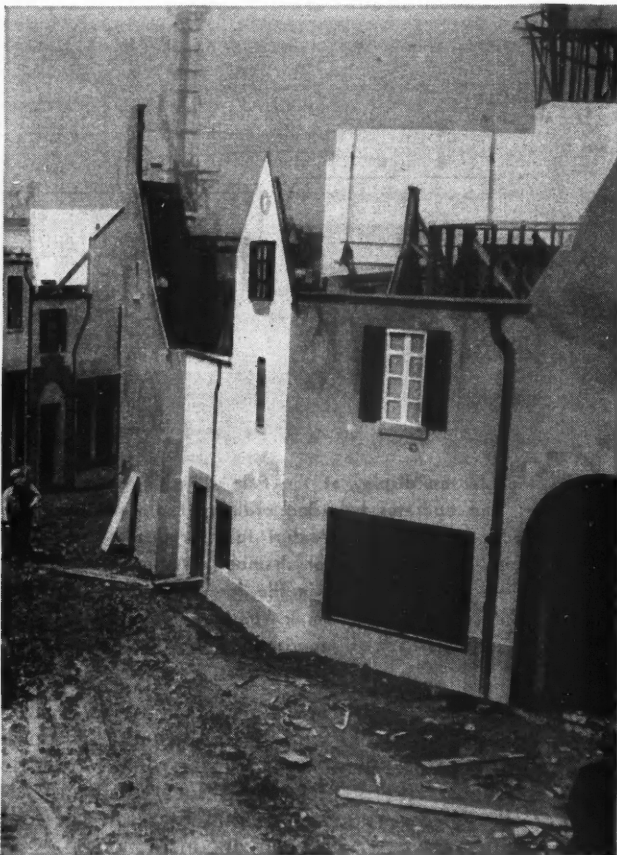
"Streets of Paris," most popular concession at the Progress World's Fair, designed by Holabird & Root, architects, and constructed by N. J. Wagner, contractor, demonstrates possibilities of giant phemaloid panel construction for quick results at low cost. Entire street front painted by Pausback Scenery Co.
