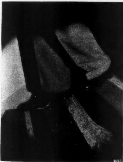
New non slip tread uses abrasive chips to prevent slipping.
