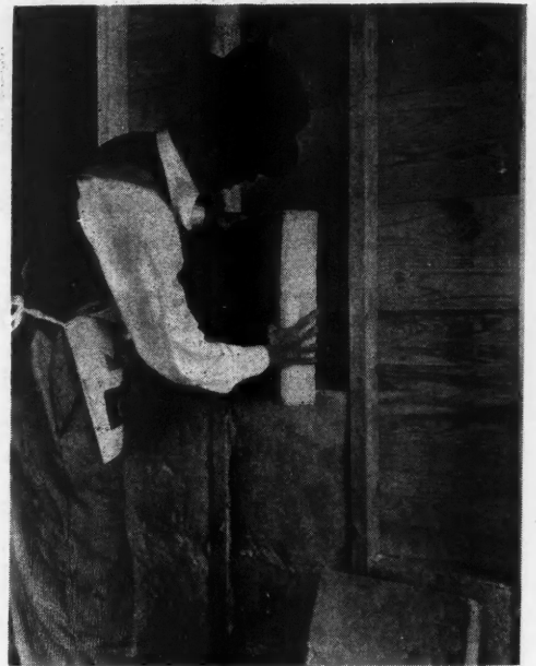
New rock wool batt comes wall thick, 15 x 18 inches in size. Weighs only 2½ pounds.
