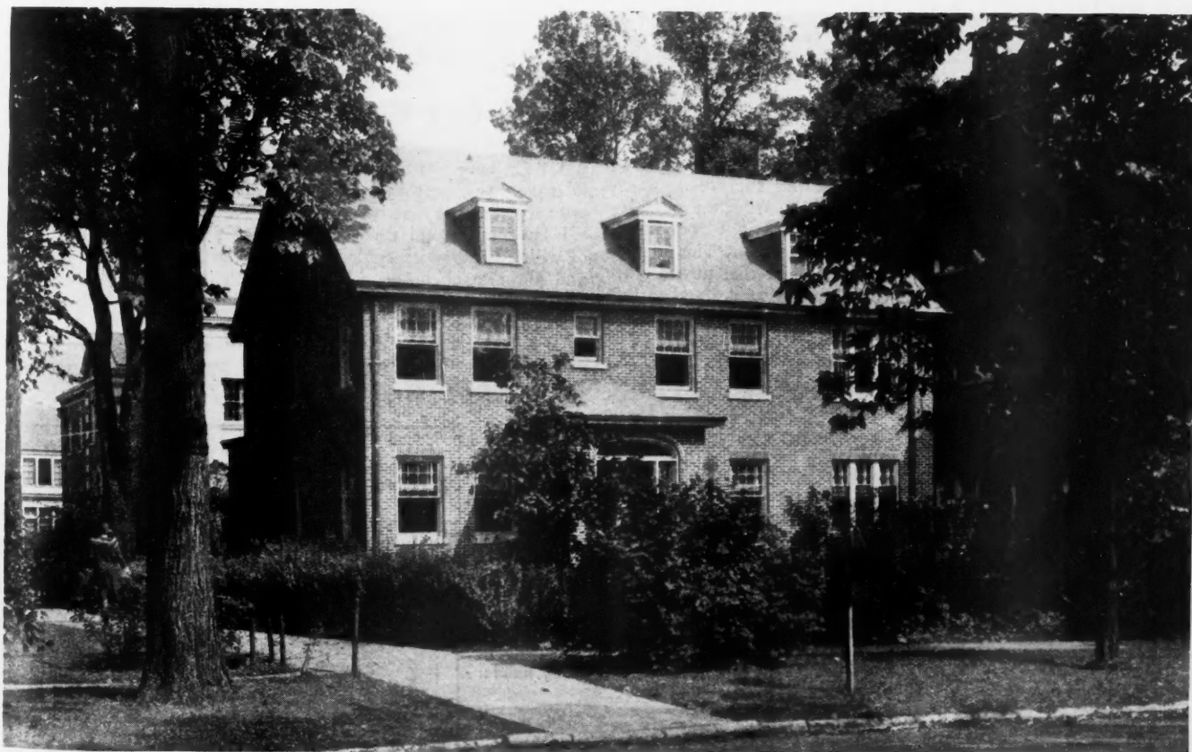
STEP 6: Finishing touches being added to completely remodeled house of E. A. Lomas, Evanston, Ill., just four months after work was started. The house is located in a valuable residential district surrounded with beautiful trees.
