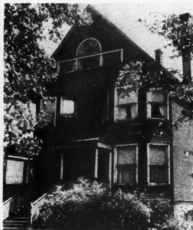
BEFORE AND AFTER views of another modernizing job sponsored by the Herald and Examiner, Chicago newspaper, in its current modernizing drive. At far left is the remodeled house with new stucco and shingle exterior.
