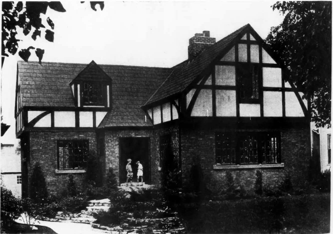
COMPLETELY MODERNIZED HOUSE which was widely publicized by Chicago newspaper and created great interest in modernizing. It is located in River Forest, a suburb, and was visited by thousands of persons. The house before modernizing is shown on opposite page.
