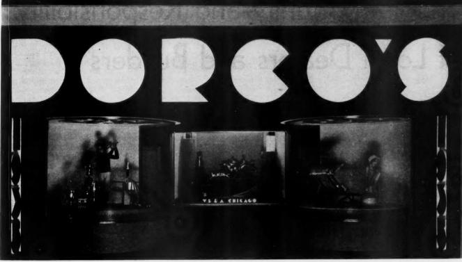
LATEST IDEAS in the use of electricity to attract attention of passersby to merchandise are shown in this modern shop. The circular windows with revolving floors are bathed in a glow of light from a battery of reflectors in the ceiling, details of which are shown below. The large electric sign across front is worked out in flashed opal glass against a black background.
