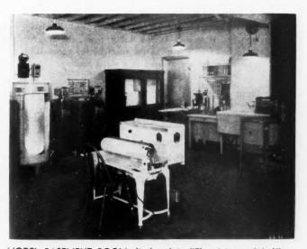
MODEL BASEMENT ROOM displayed in "Electricity at Work" exhibit at World's Fair, showing complete modern home laundry, water softening equipment, electric water heater, complete air conditioning.
