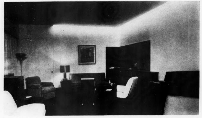
CONCEALED COVE LIGHTING which is detailed below is the feature of this modern living room. This provides efficient illumination and gives tonality to the walls through use of various shades and colors, which may be adapted to the mood of the occupant.
