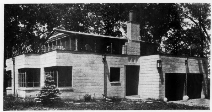
THIS COMFORTABLY MODERN HOME IS BUILT of permanent, time-tested materials that lend themselves admirably to this new type of design. Concrete units, given only a finish of white portland cement paint, were used. It is located in Des Moines, Ia., and Amos B. Emery is the architect. Cost of construction was surprisingly low.
