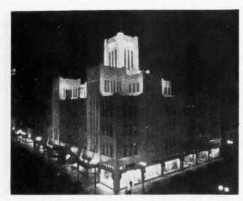
Wise Brothers Department Store, Los Angeles, California, a typical set-back type of building which is especially suitable for flood lighting. Flood lighting projectors are mounted on the building entirely concealed from view.
