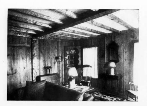
WALLS ARE COVERED with cedar shingles spaced 5" to the weather; asbestos shingles are used on roofs. Hand hewn pine timbers are used in the living room secured with hand made dowels. Side walls were sheathed with varying widths of  $7/_8$ " pine and joints covered with  $1/_2$ " strip moulding with a small bead on each edge for decoration.
