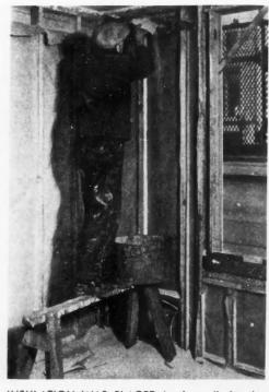
INSULATION WAS PLACED in the walls by the contractor's workman. A treated sawdust was used to provide both insulation and fire protection.
