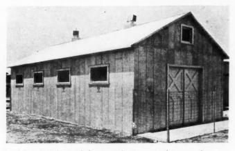
World's Fair Building of sheet metal units erected in one afternoon, using construction shown in details below.
