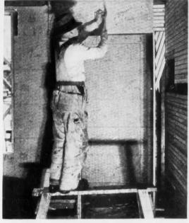
NEW INSULATING LATH PLASTER BASE was put on over old wood lath after old plaster had been torn away. Many new and interesting materials and methods were demonstrated by Contractor Griffith. At left is shown how the floor plan of the renovized house looked.
