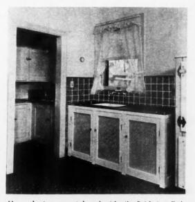
New asbestos cement board with tile finish installed in modern kitchen.
