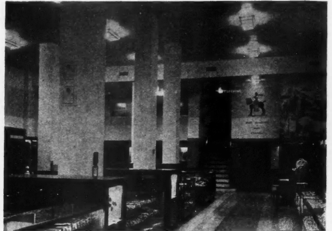
MODERN STORE INTERIOR has latest lighting equipment. Intensity of light is controlled by "electric eye" in pillar.
