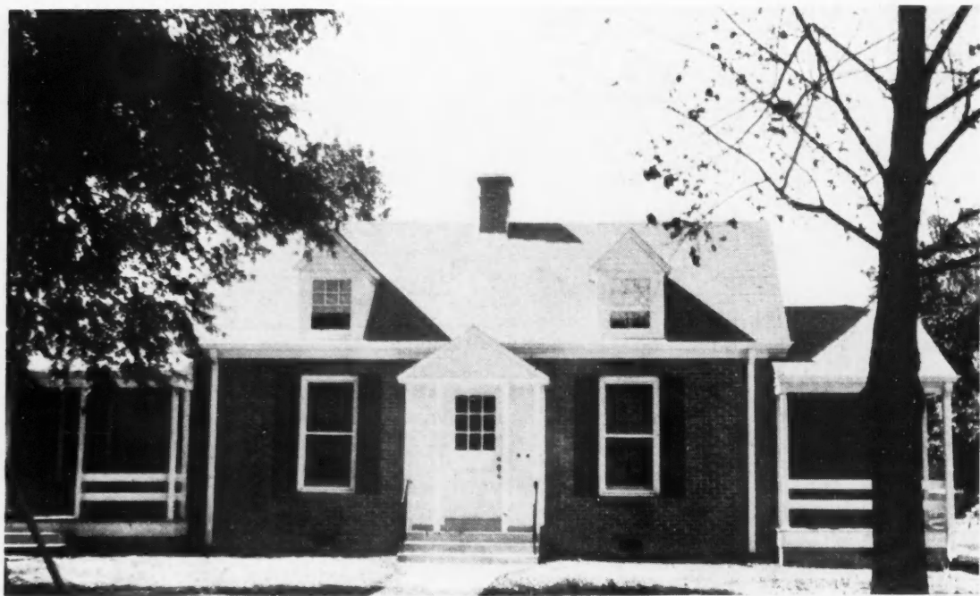
FRONT VIEW of the remodeled duplex apartment at Corinth, Miss. Both apartments were rented before remodeling was completed. Thomas H. Johnston, Jr., Architect.
