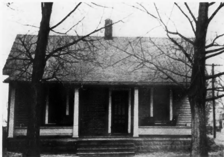
HERE IS THE FRONT VIEW of the old structure—a typical old house with old fashioned plumbing and heating, and no architectural style.
