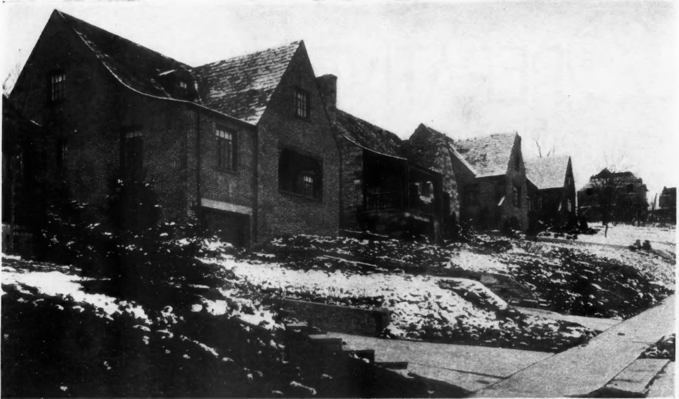
ROW OF "Ab" Young's houses on Mayfair Drive, Mt. Lebanon (Pittsburgh) built and sold this winter at from $11,000 to $16,000. Brick and stone veneer, asbestos colorblend shingle roofs and steel supported concrete first floors are favored. Real estate salesmen find a brisk demand for such well built homes.
