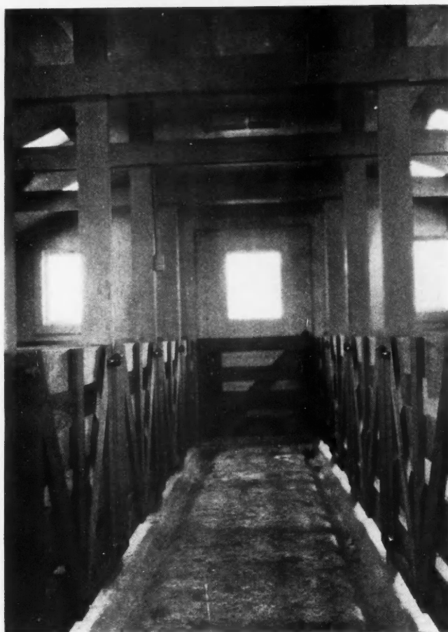
FEED ALLEY in Hog House Showing Drain Troughs, Pen Gates and Roof Framing. The direct sunshine from the battery of 12 roof windows, 6 on each side, warms and sweetens the pens for early spring farrowing.
