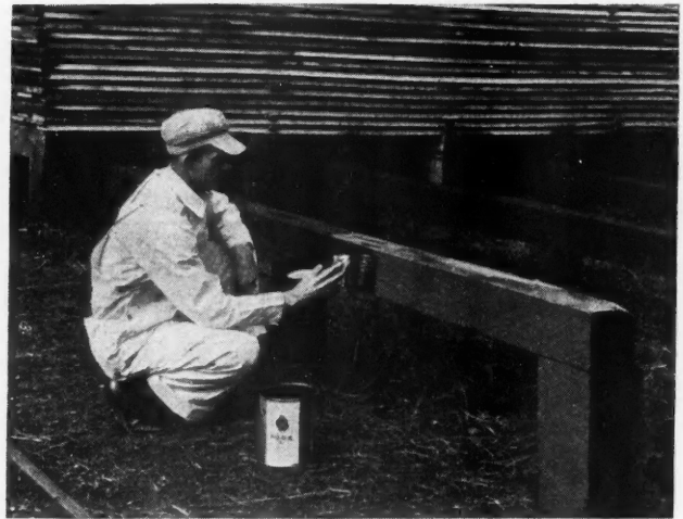
Applying termite protection
